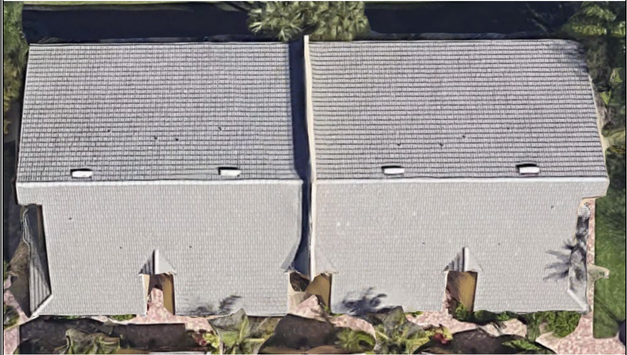
View of roof geometry (per question 5).
