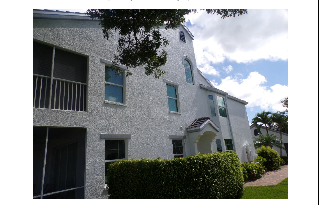
View of typical glazed openings (per question 7).
