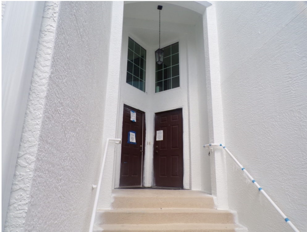
View of non-glazed openings (per question 7).
