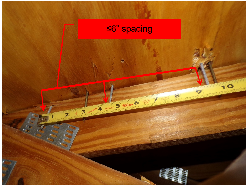
View of re-nailing pattern (per question 3).
