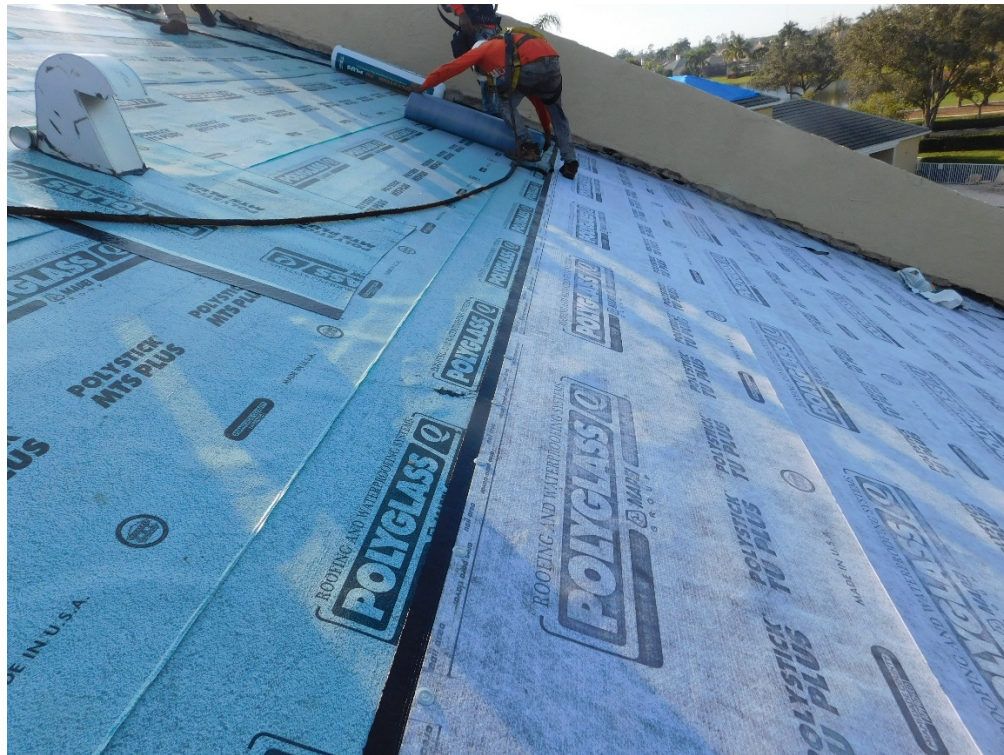
View of self-adhering roofing underlayment (per question 6).
