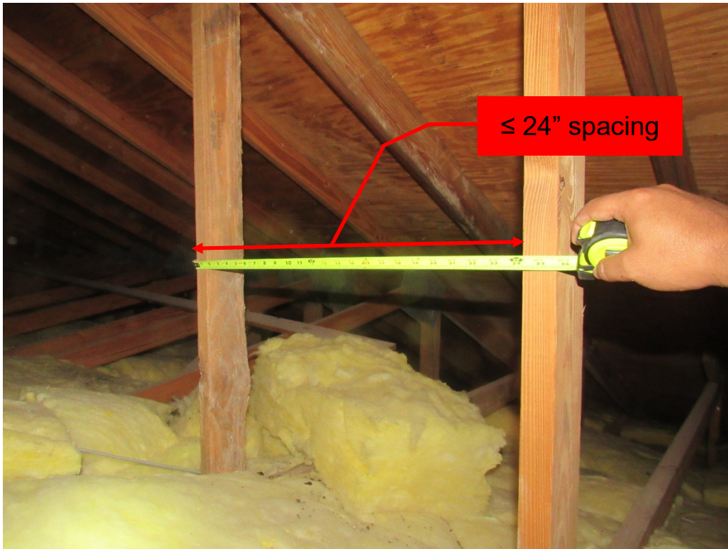
View of truss spacing (per question 3).
