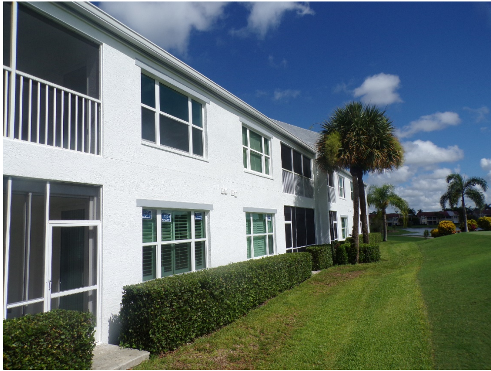
View of typical glazed openings (per question 7).
