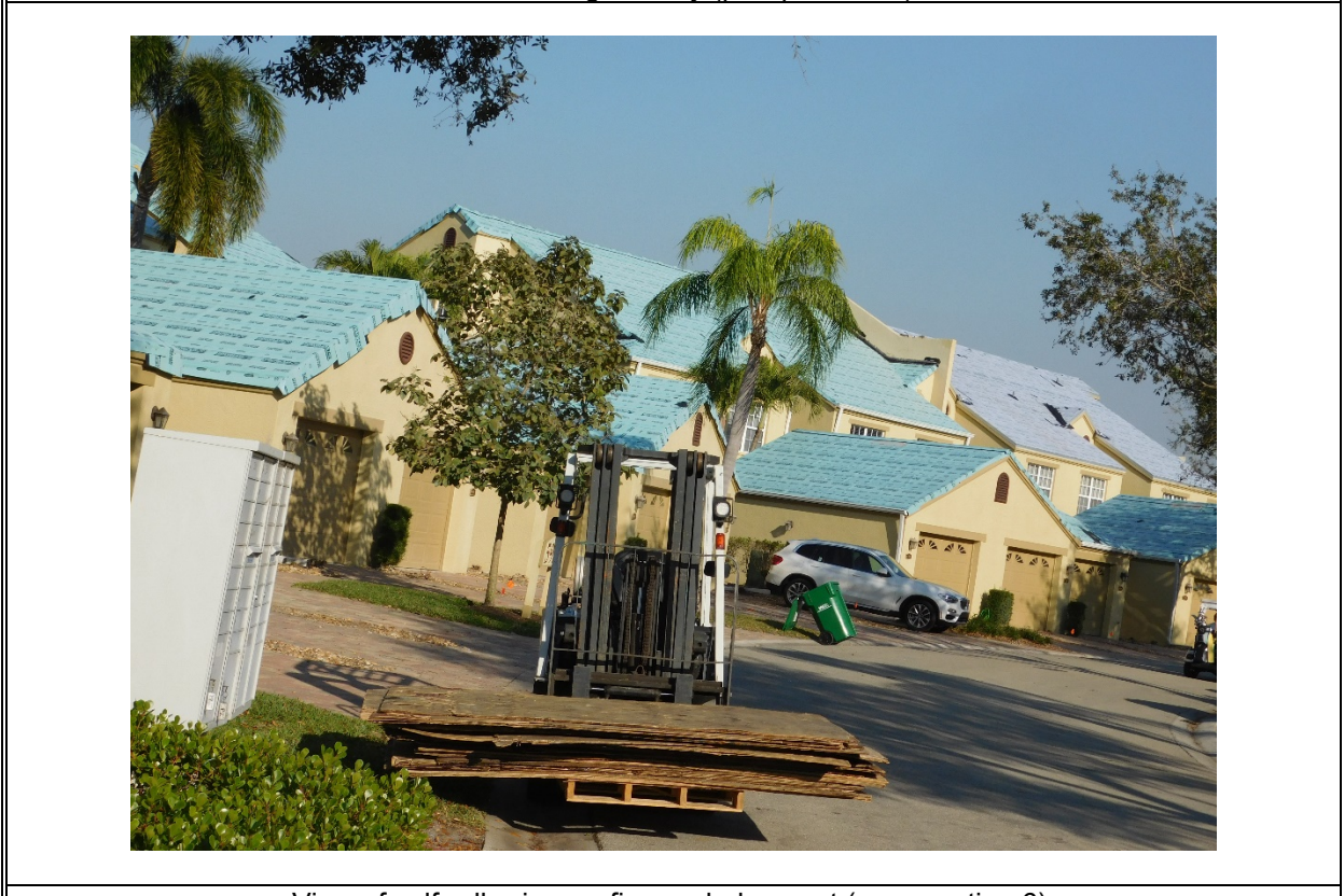
View of self-adhering roofing underlayment (per question 6).
