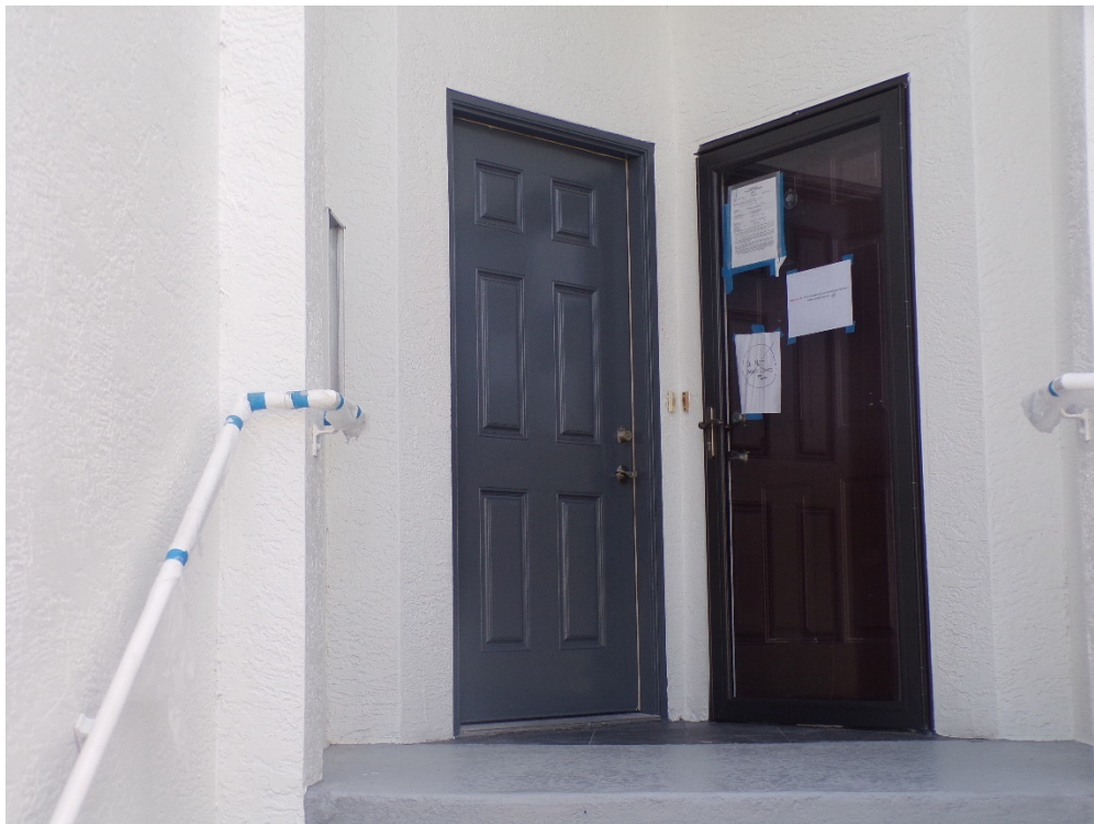
View of non-glazed openings (per question 7).
