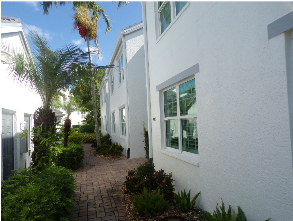
View of typical glazed openings (per question 7).
