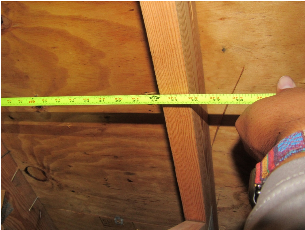
View of truss spacing (per question 3).
