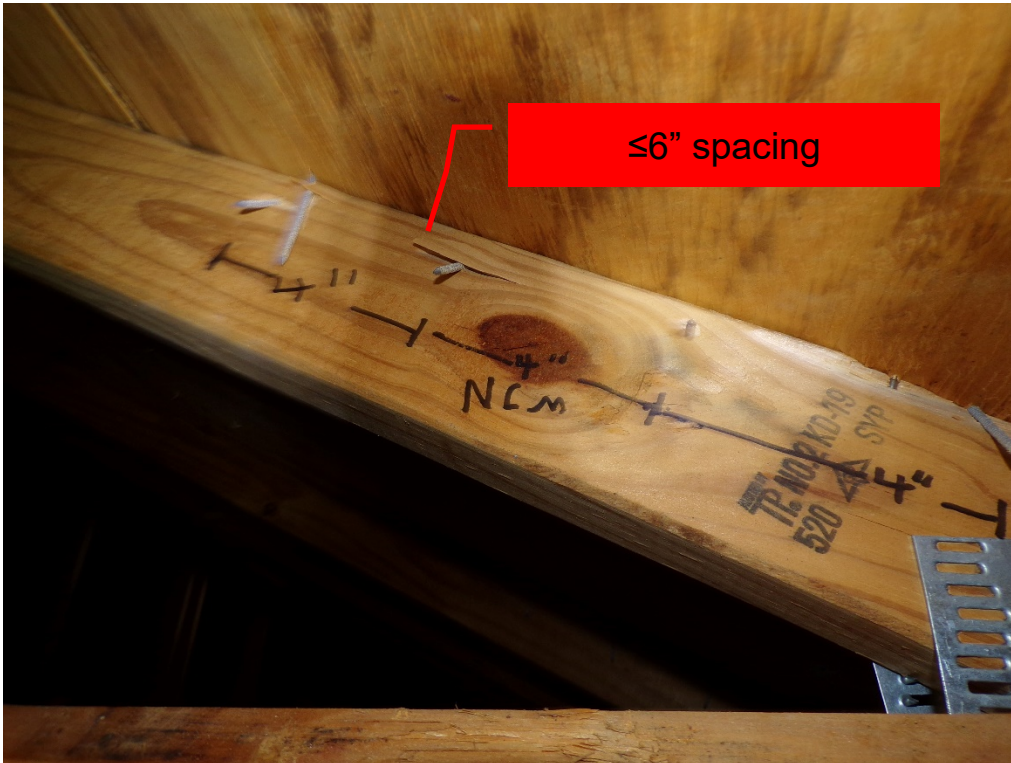
View of re-nailing pattern (per question 3).
