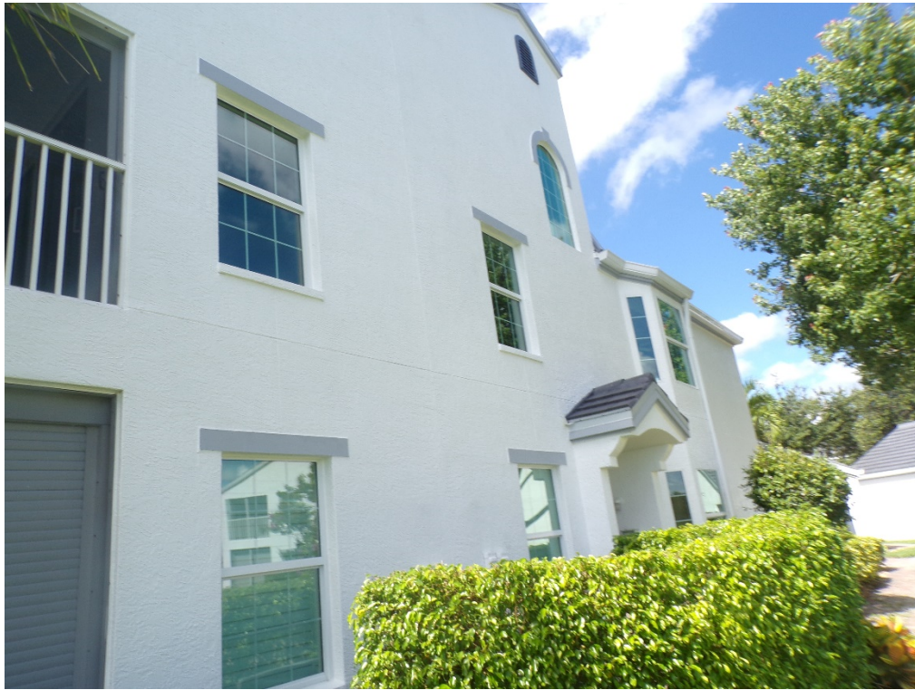
View of typical glazed openings (per question 7).
