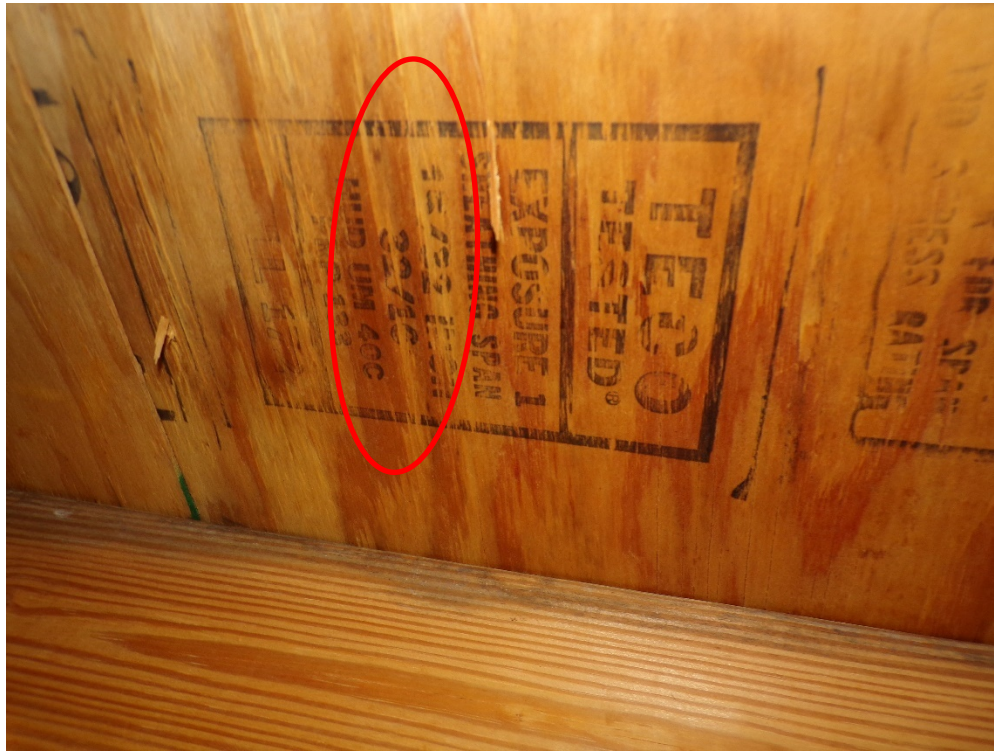
View of existing plywood sheathing thickness (15/32) per question 3.
