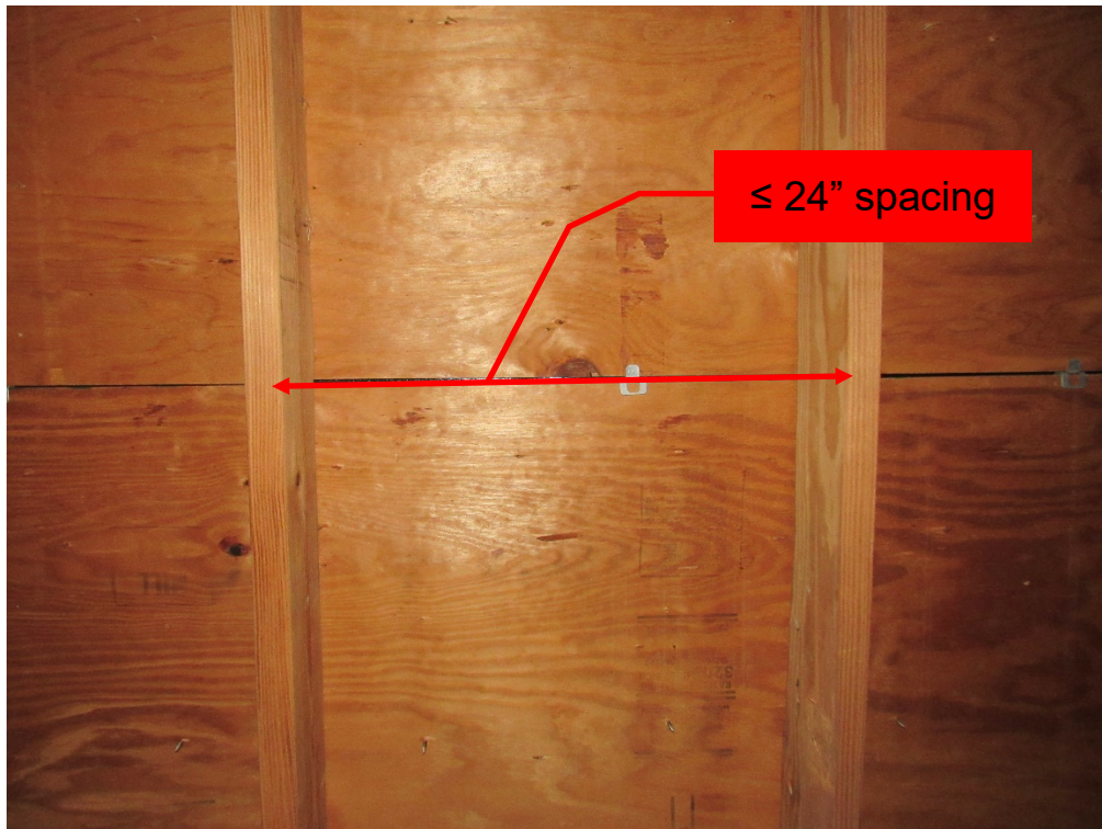
View of truss spacing (per question 3).
