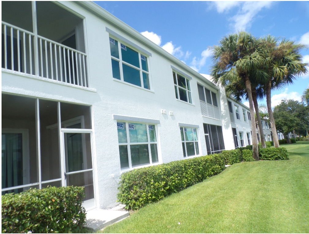
View of typical glazed openings (per question 7).
