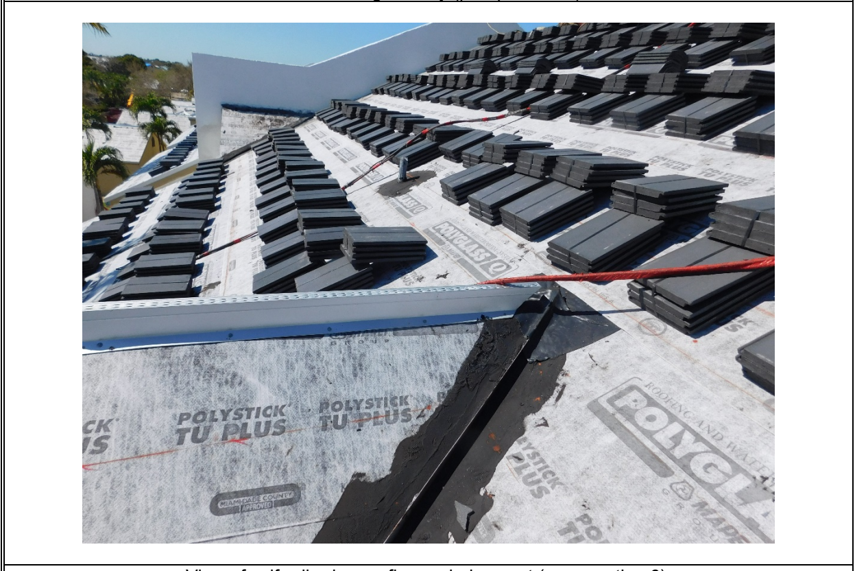
View of self-adhering roofing underlayment (per question 6).
