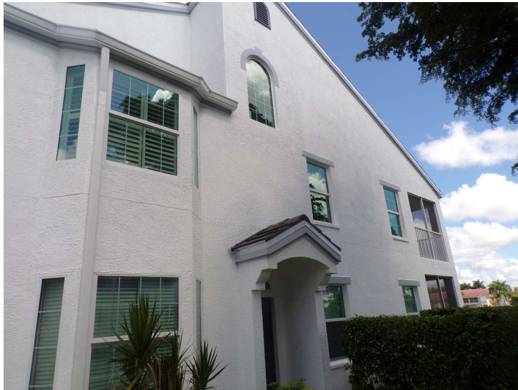
View of typical glazed openings (per question 7).
