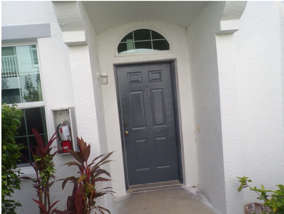
View of non-glazed openings (per question 7).
