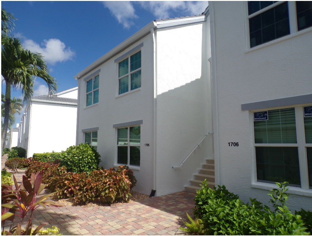
View of typical glazed openings (per question 7).
