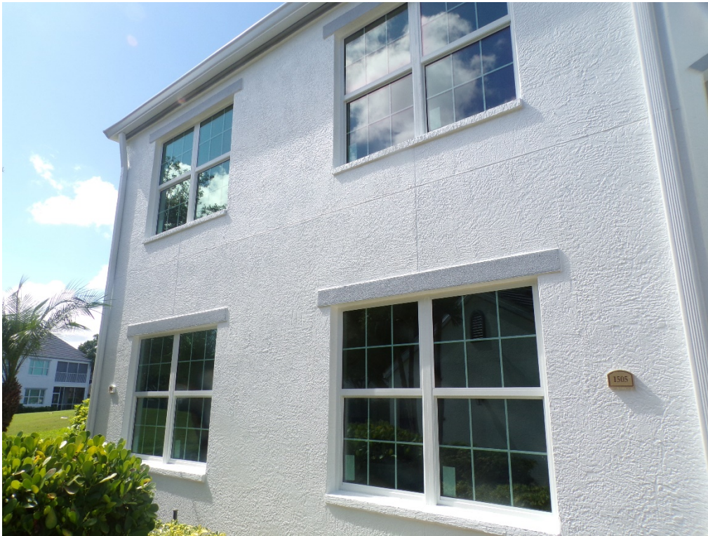
View of typical glazed openings (per question 7).
