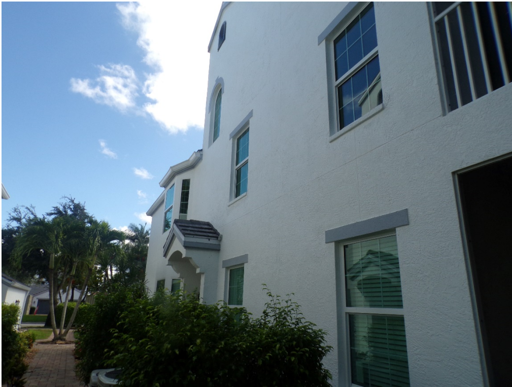
View of typical glazed openings (per question 7).
