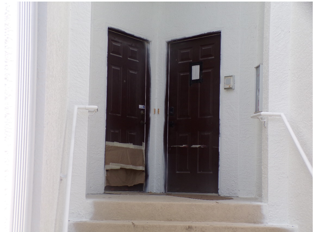
View of non-glazed openings (per question 7).
