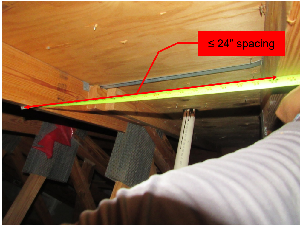
View of truss spacing (per question 3).
