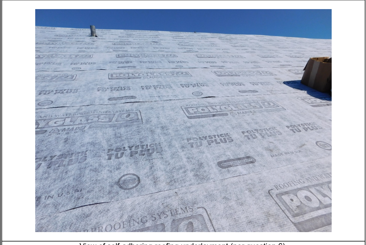
View of self-adhering roofing underlayment (per question 6).
