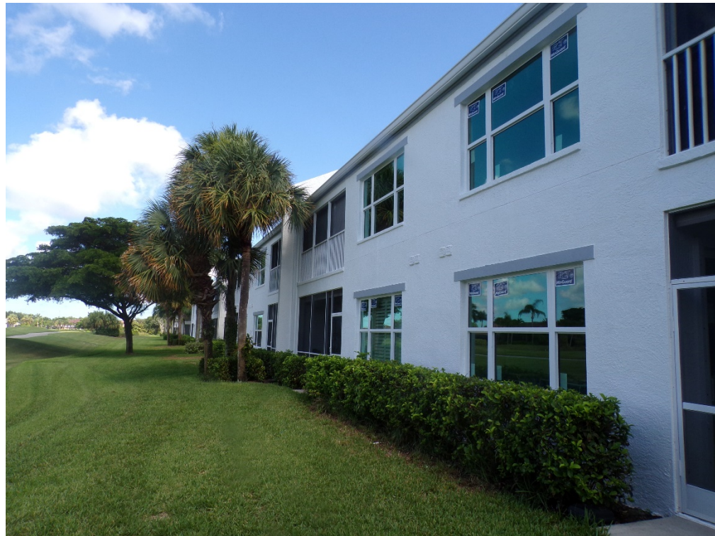
View of typical glazed openings (per question 7).
