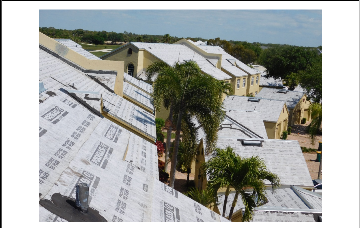
View of self-adhering roofing underlayment (per question 6).
