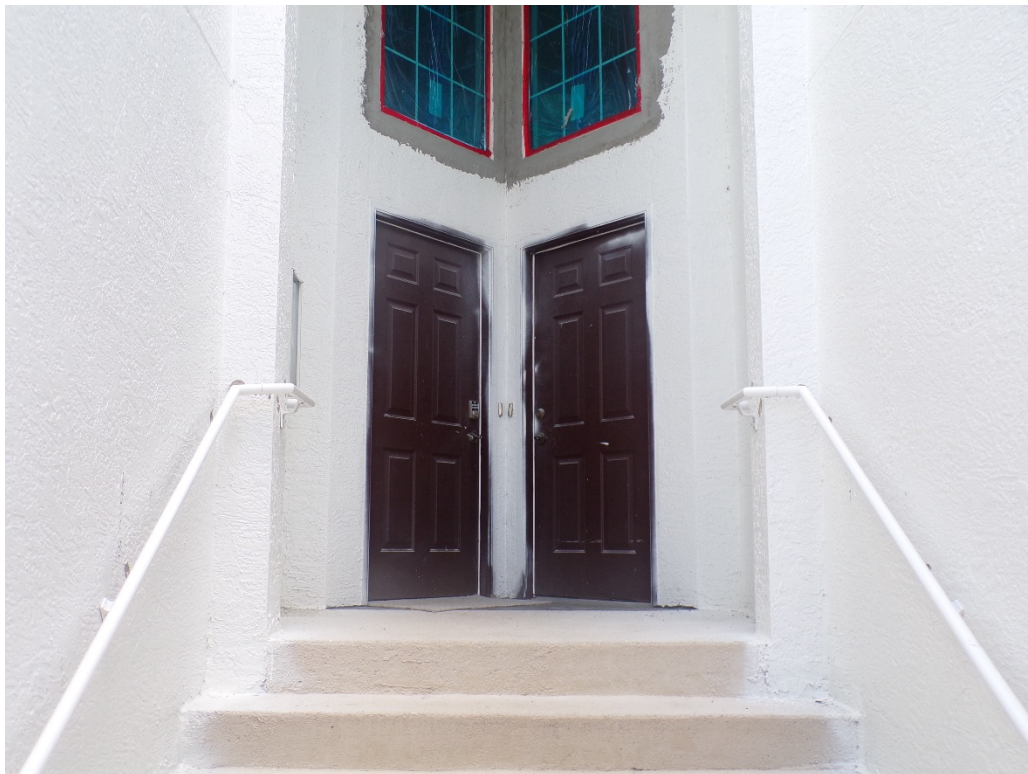
View of non-glazed openings (per question 7).
