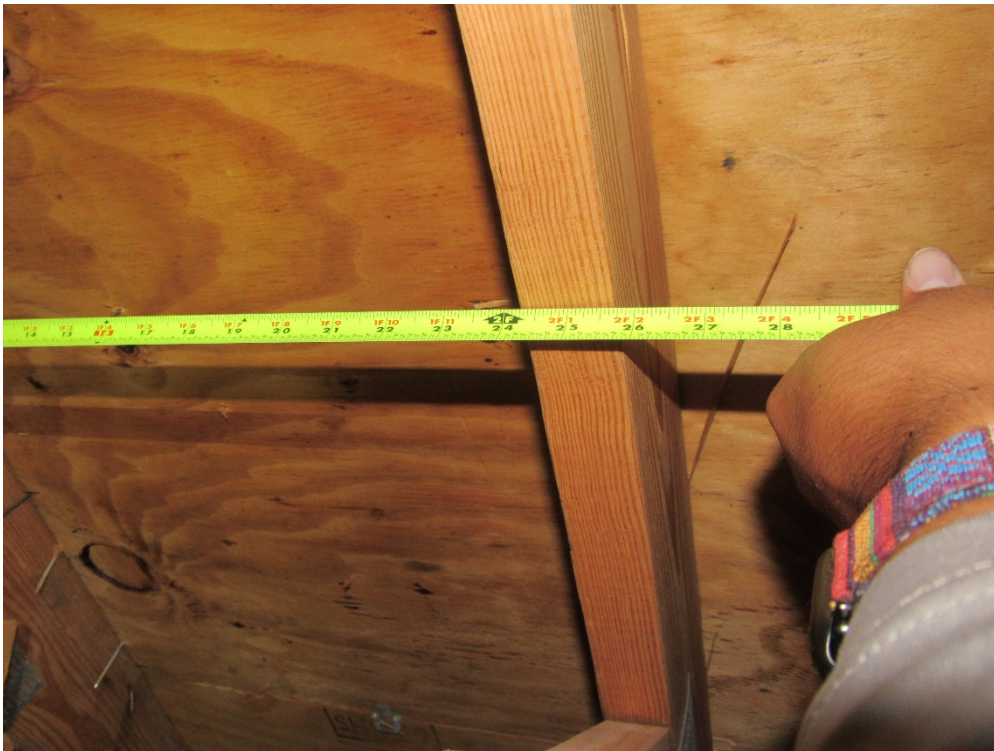
View of truss spacing (per question 3).
