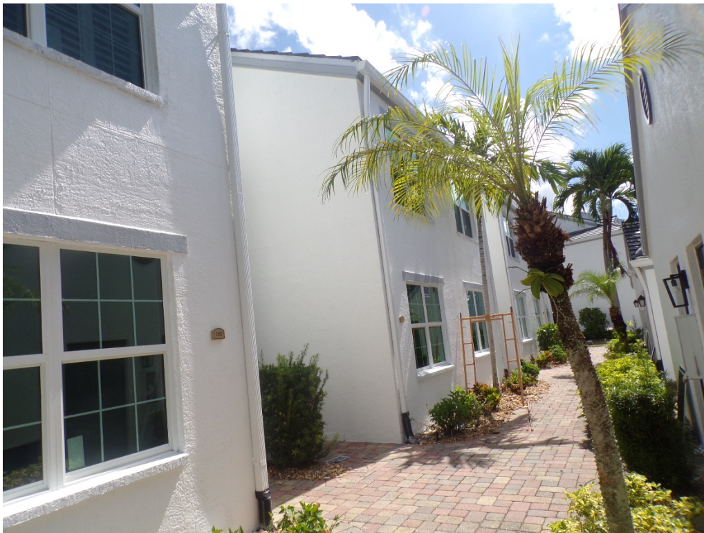
View of typical glazed openings (per question 7).
