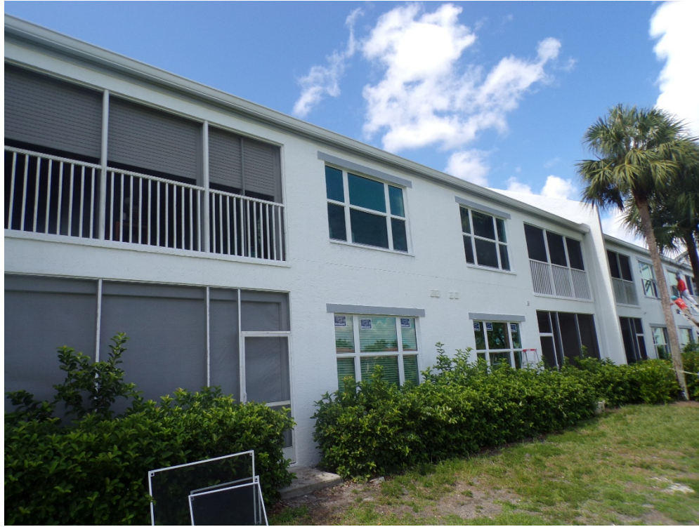
View of typical glazed openings (per question 7).
