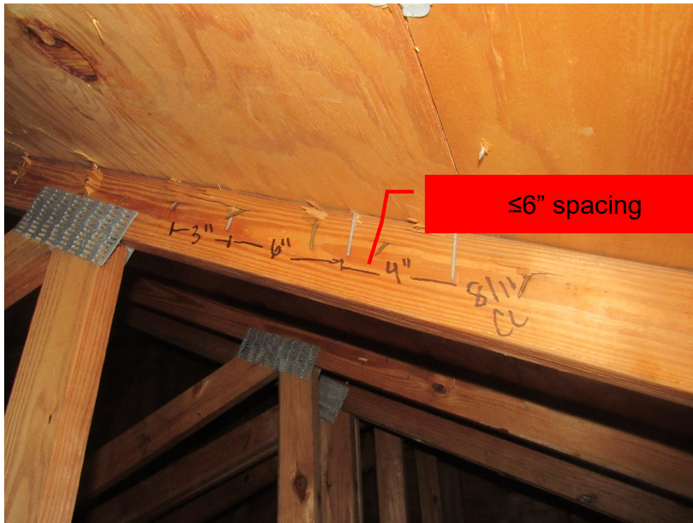
View of re-nailing pattern (per question 3).
