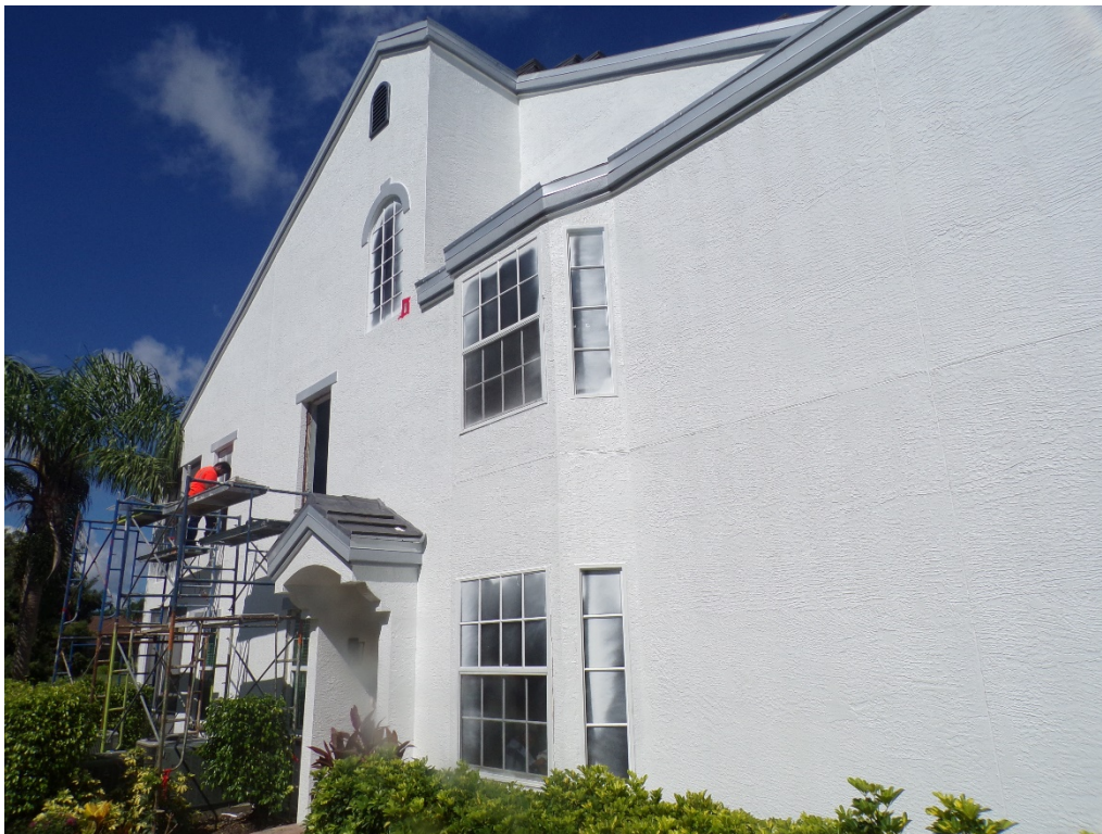
View of typical glazed openings (per question 7).
