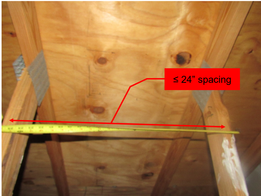
View of truss spacing (per question 3).
