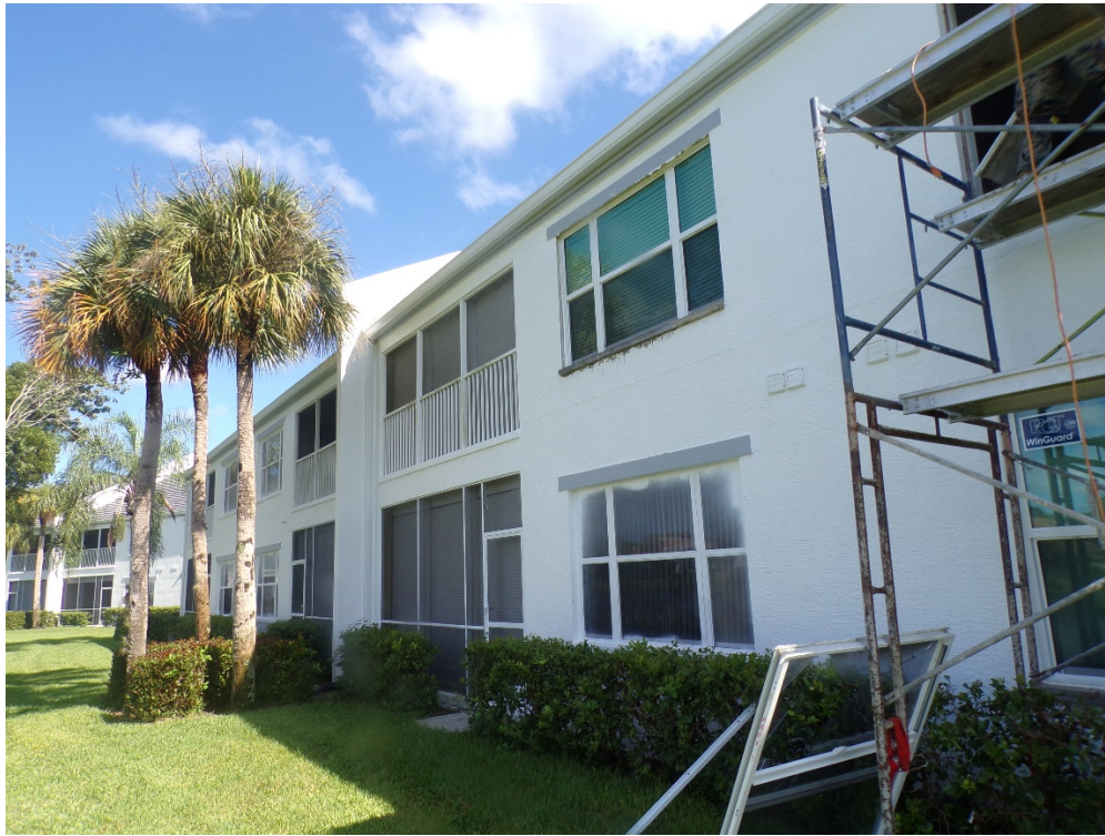
View of typical glazed and non-glazed openings (per question 7).
