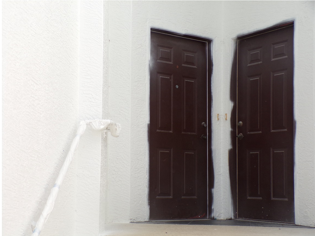
View of typical non-glazed openings (per question 7).
