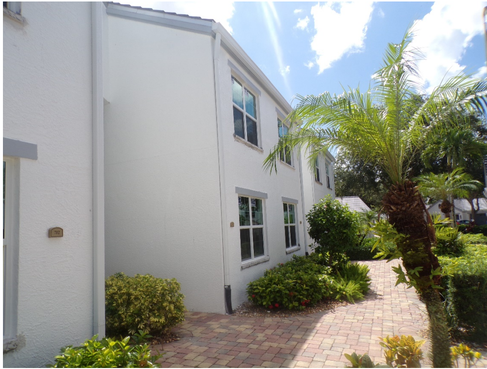
View of typical glazed openings (per question 7).
