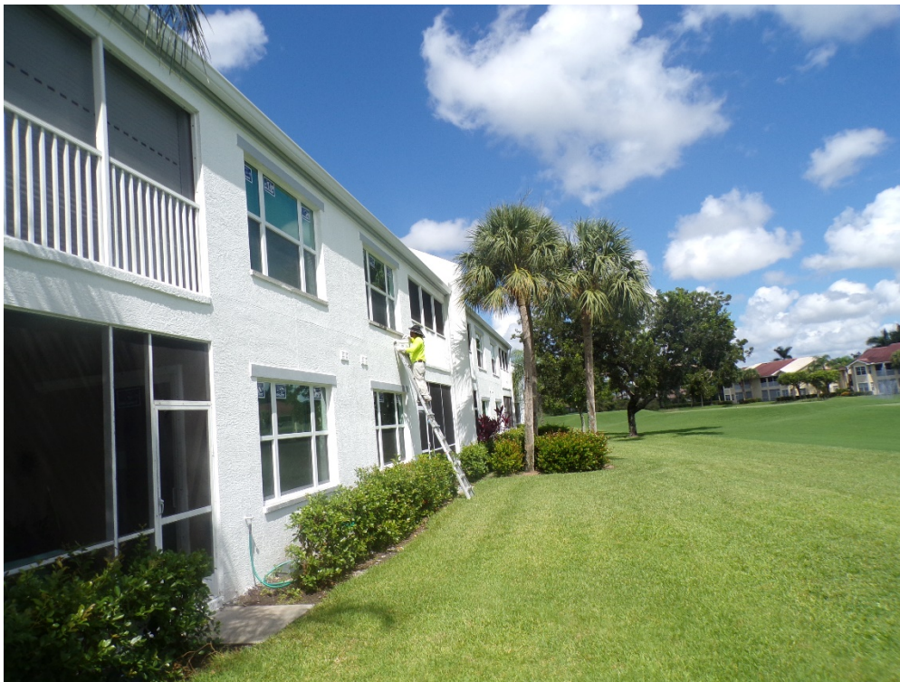
View of typical glazed openings (per question 7).
