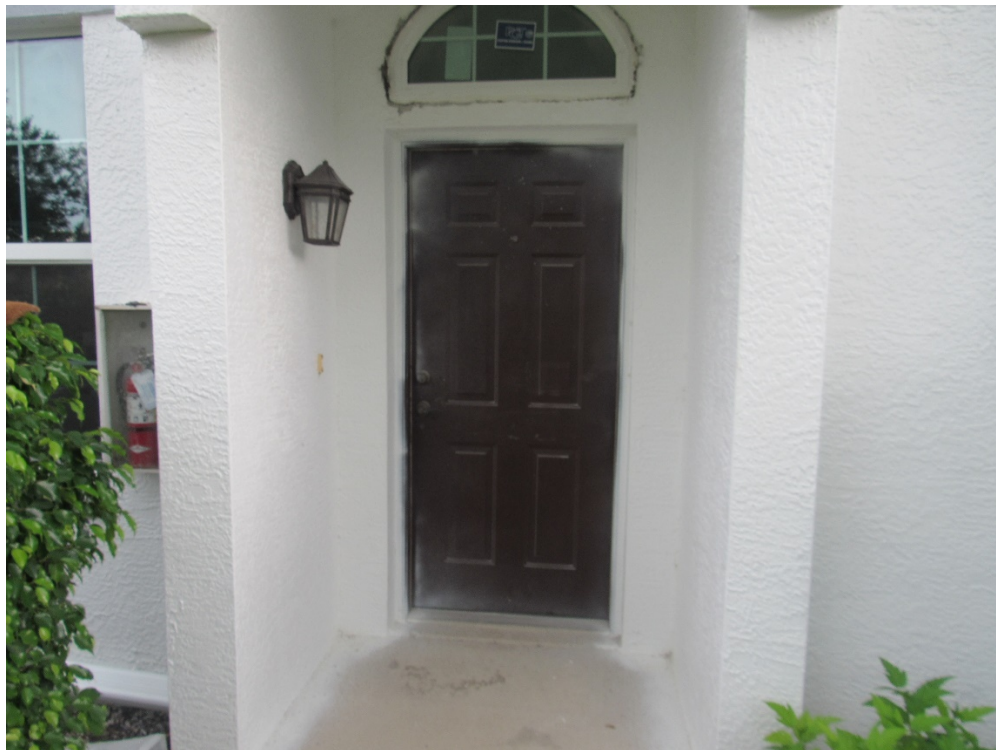
View of non-glazed openings (per question 7).
