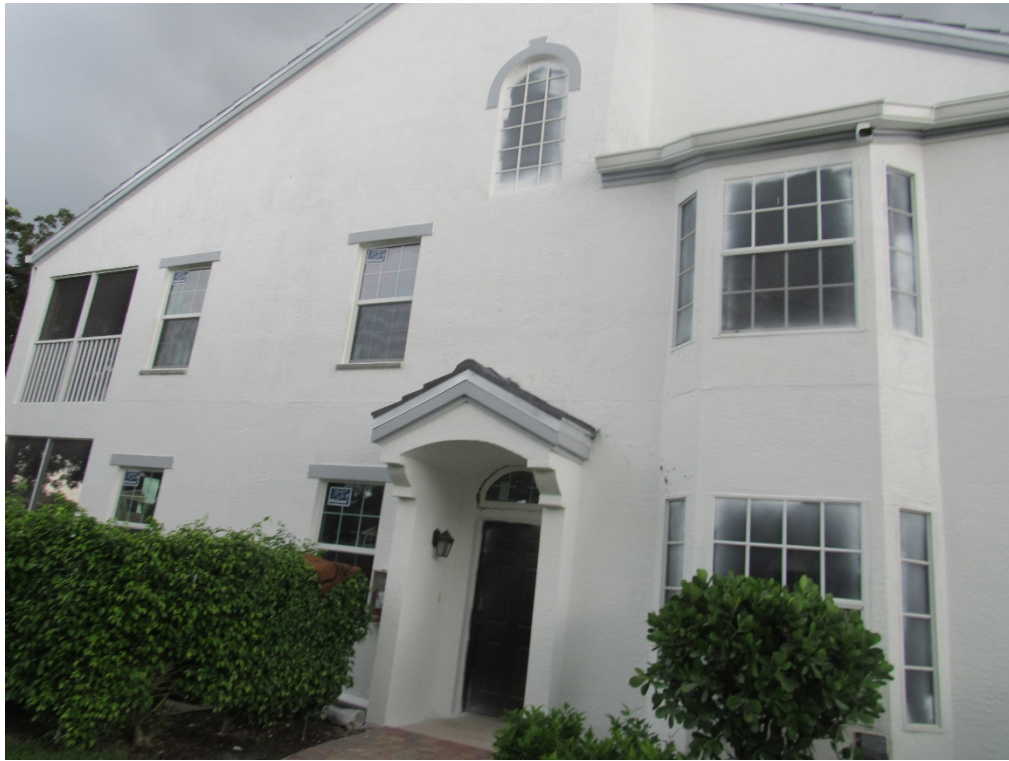
View of typical glazed openings (per question 7).
