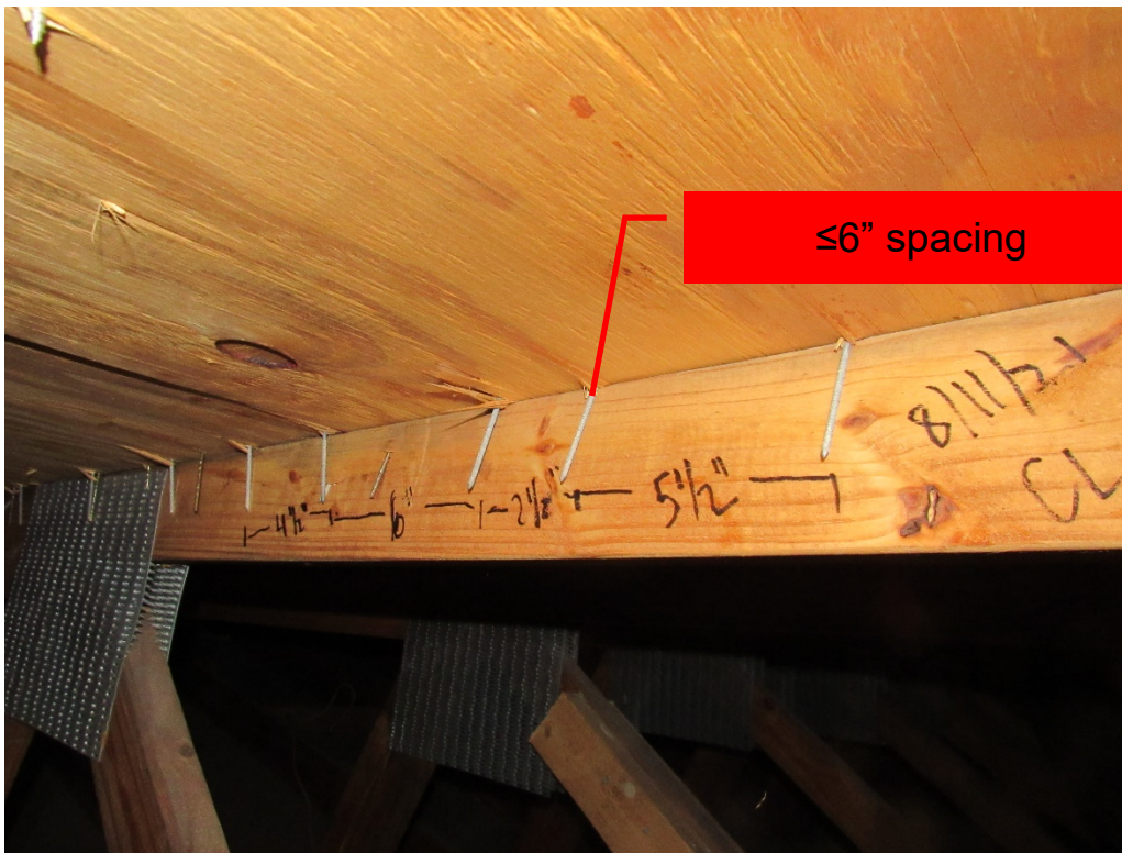
View of re-nailing pattern (per question 3).
