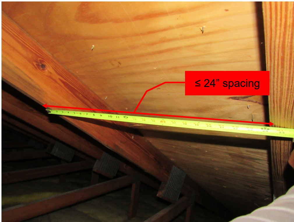
View of truss spacing (per question 3).
