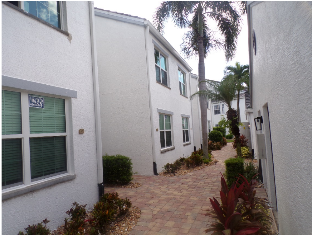
View of typical glazed openings (per question 7).
