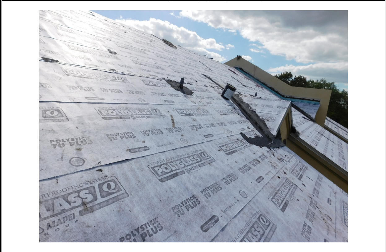
View of self-adhering roofing underlayment (per question 6).
