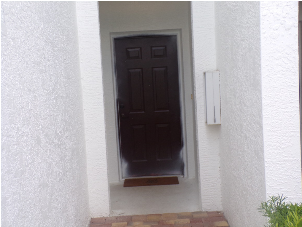
View of non-glazed openings (per question 7).
