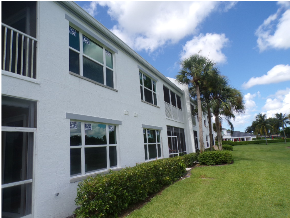
View of typical glazed openings (per question 7).
