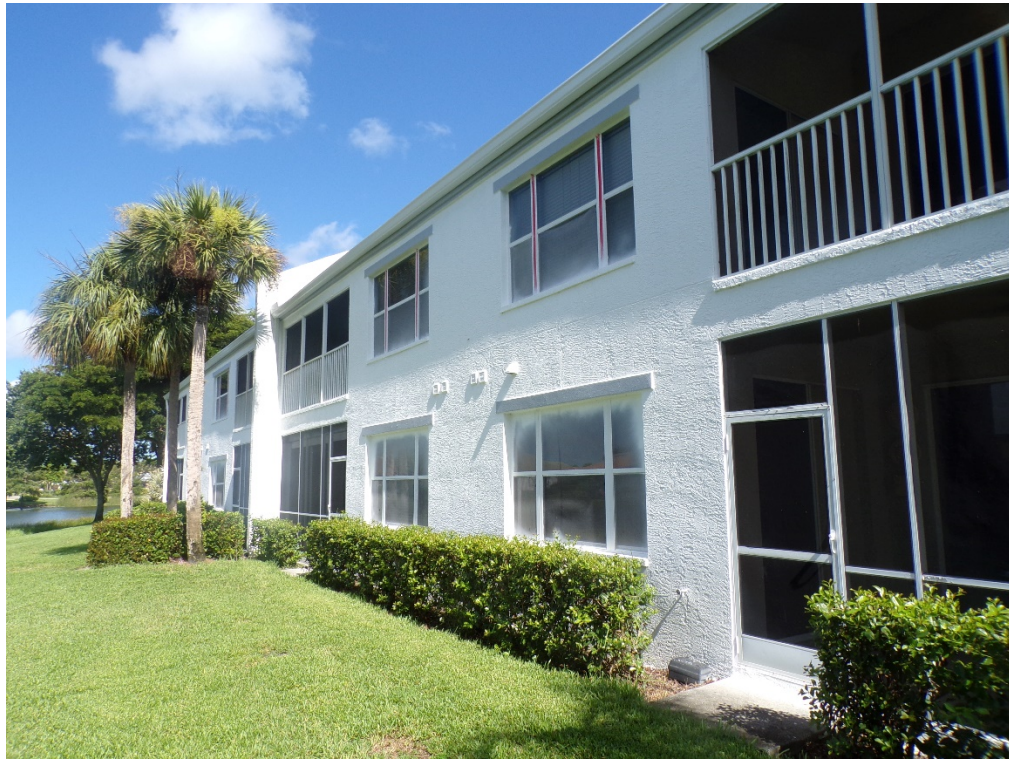
View of typical glazed openings (per question 7).
