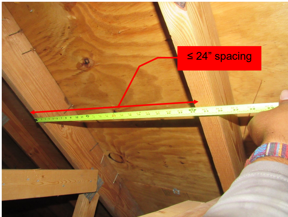
View of truss spacing (per question 3).
