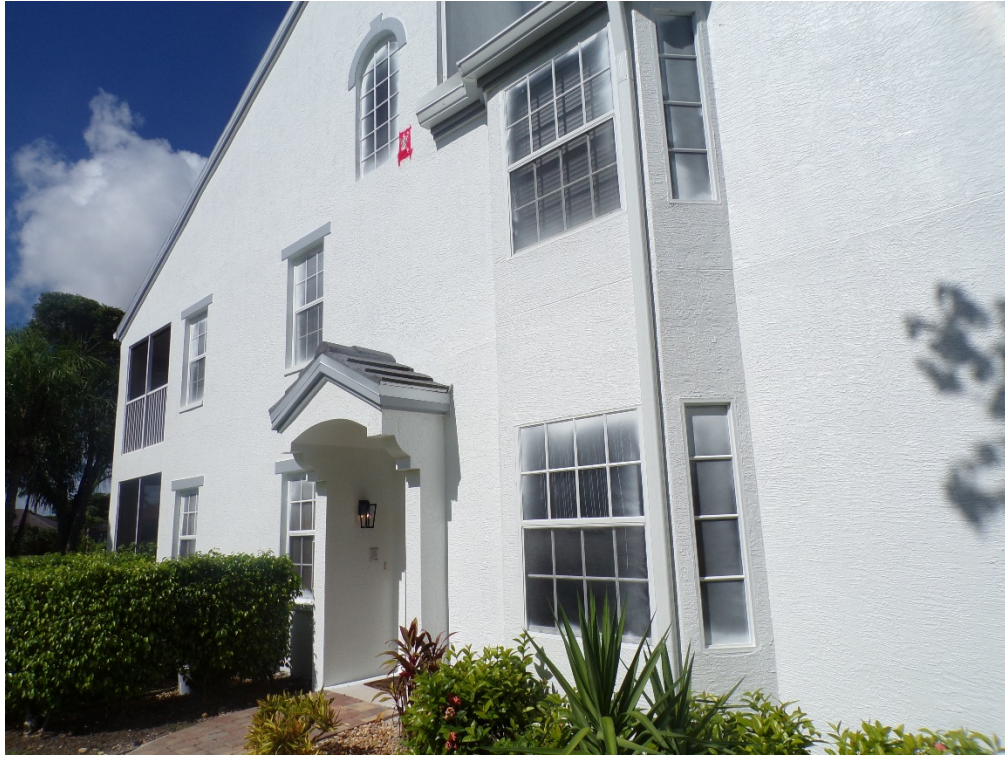
View of typical glazed openings (per question 7).
