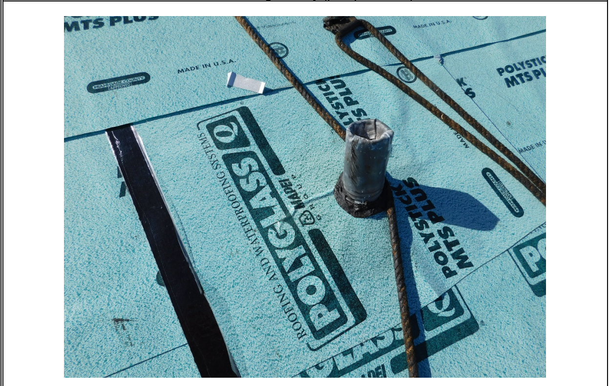
View of self-adhering roofing underlayment (per question 6).
