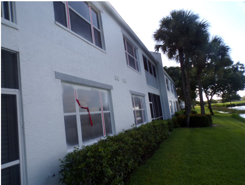
View of typical glazed openings (per question 7).
