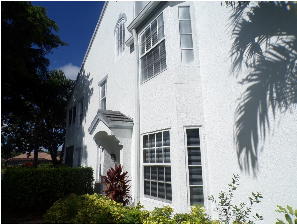
View of typical glazed openings (per question 7).
