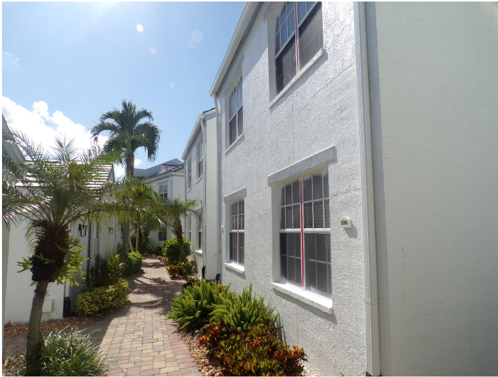
View of typical glazed openings (per question 7).
