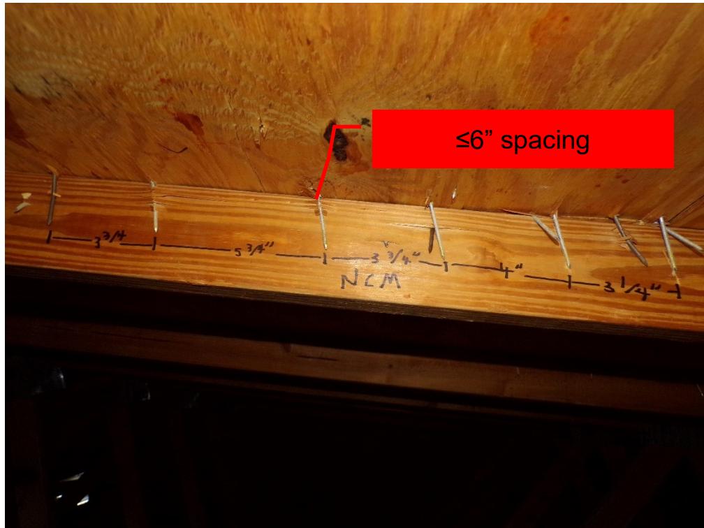
View of re-nailing pattern (per question 3).
