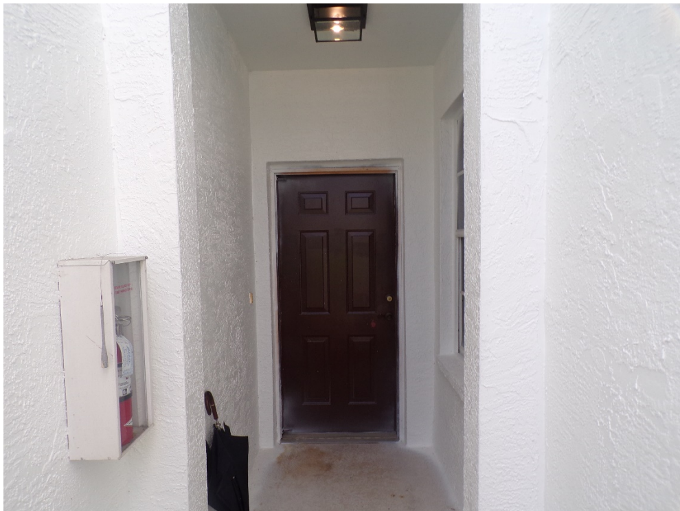
View of typical non-glazed openings (per question 7).
