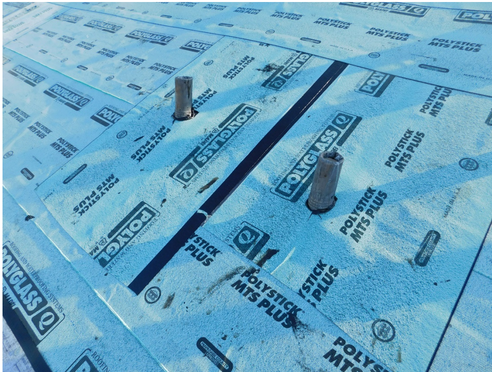
View of self-adhering roofing underlayment (per question 6).
