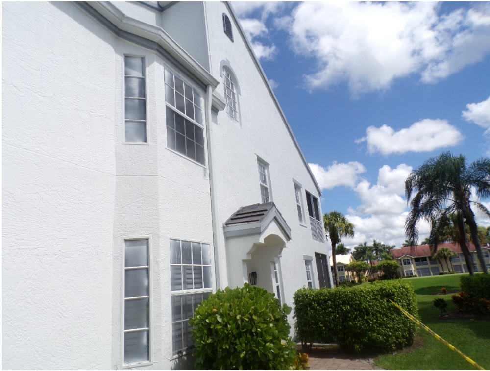
View of typical glazed openings (per question 7).
