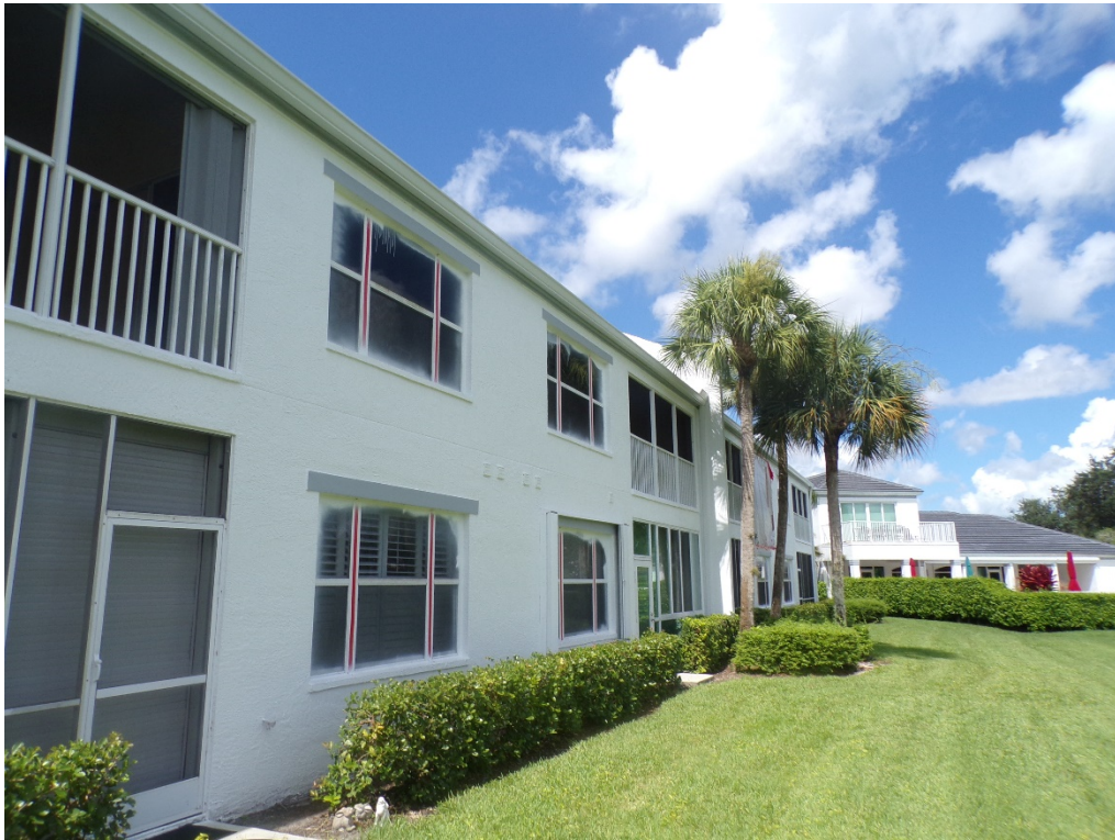
View of typical glazed openings (per question 7).
