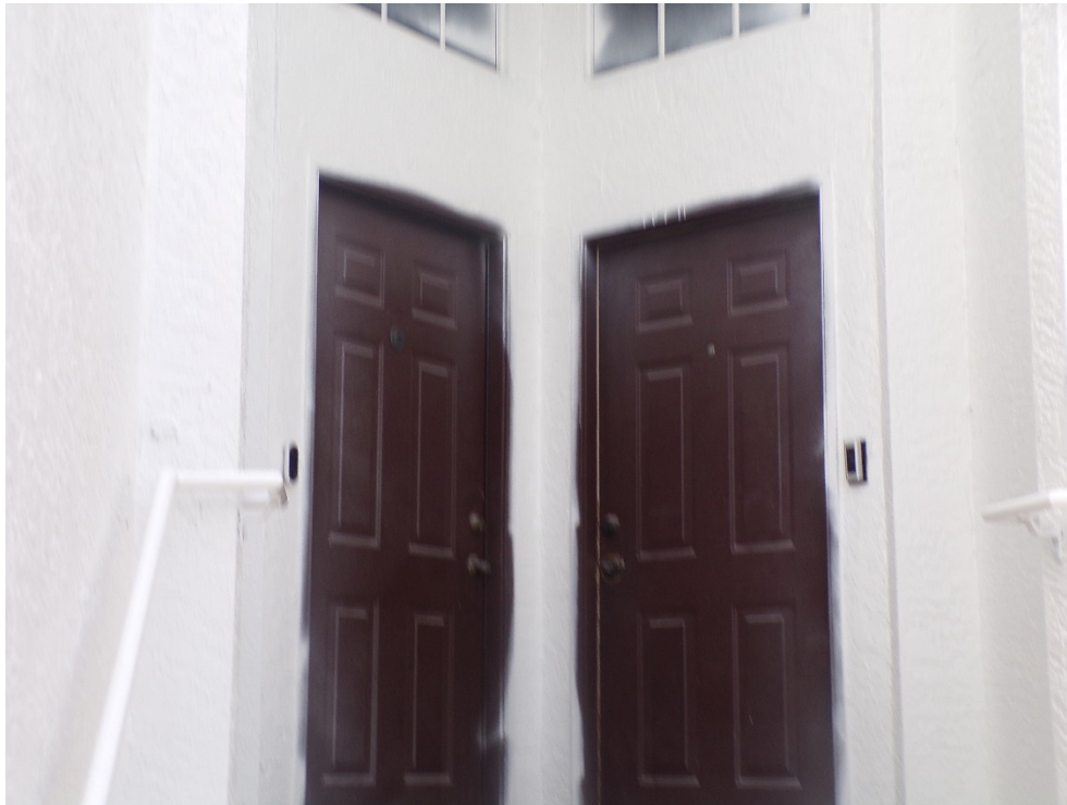
View of typical non-glazed openings (per question 7).
