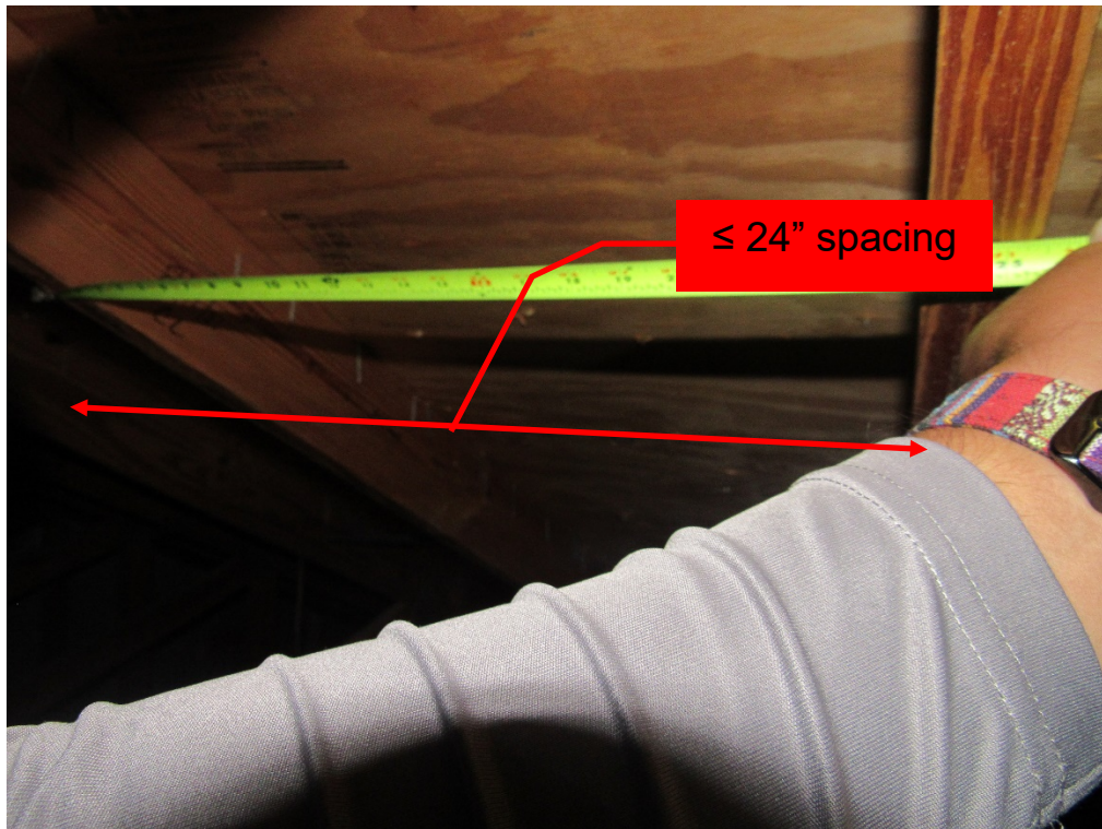
View of truss spacing (per question 3).
