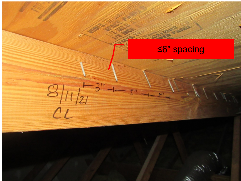
View of re-nailing pattern (per question 3).
