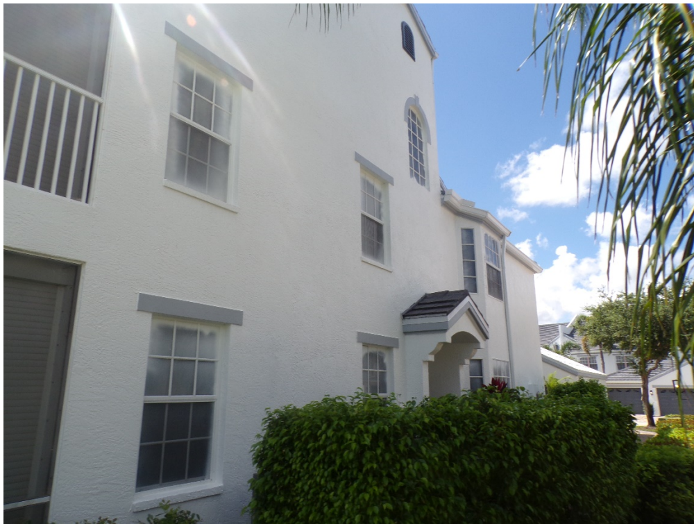
View of typical glazed openings (per question 7).
