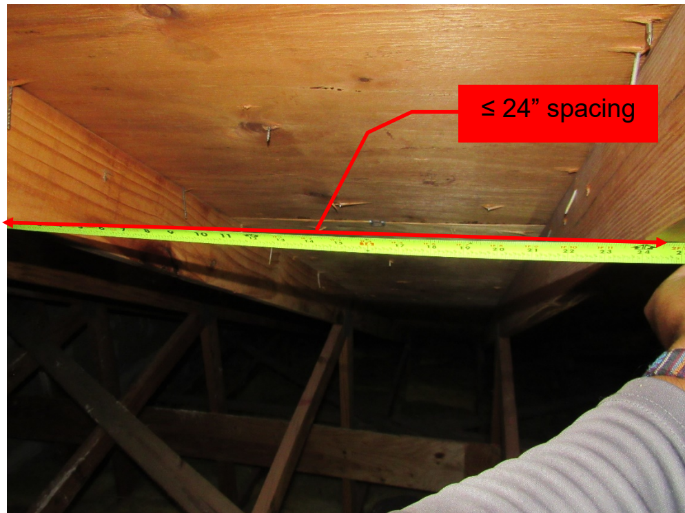
View of truss spacing (per question 3).
