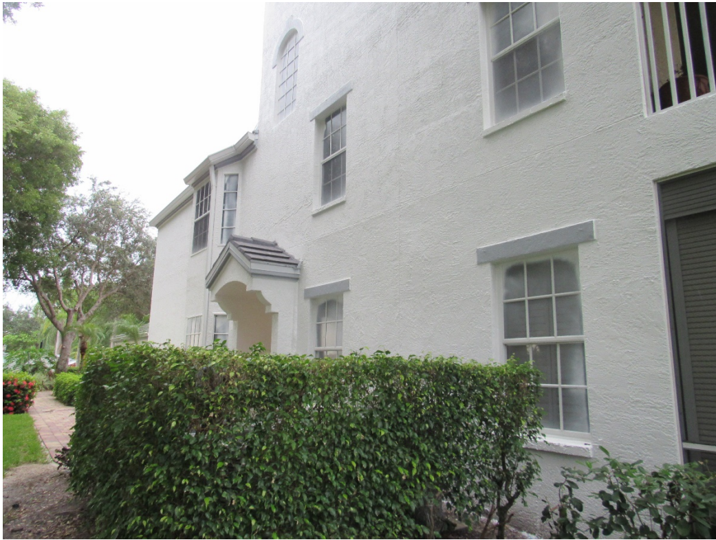
View of typical glazed openings (per question 7).
