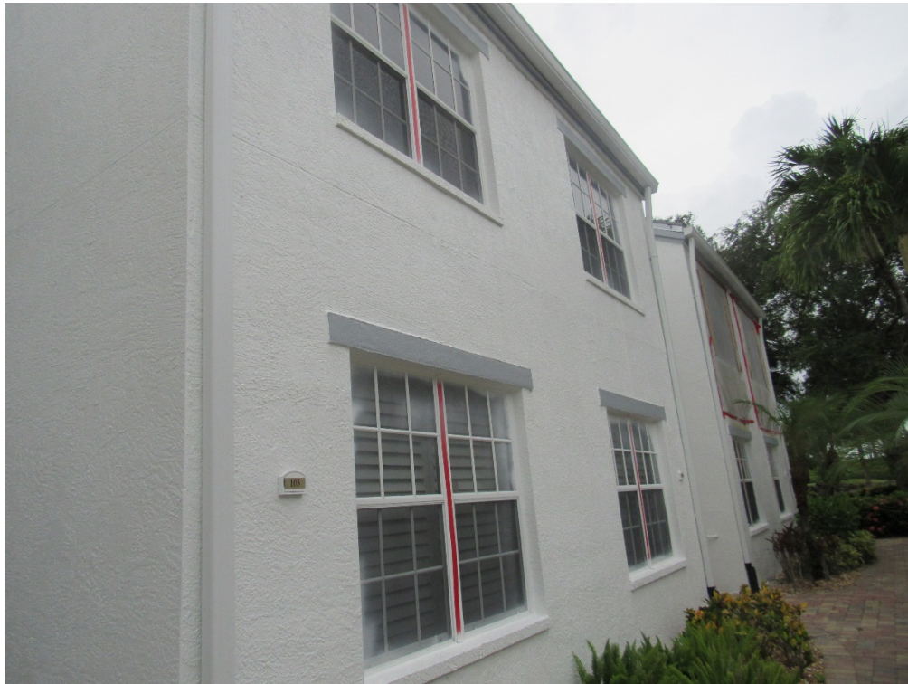
View of typical glazed openings (per question 7).
