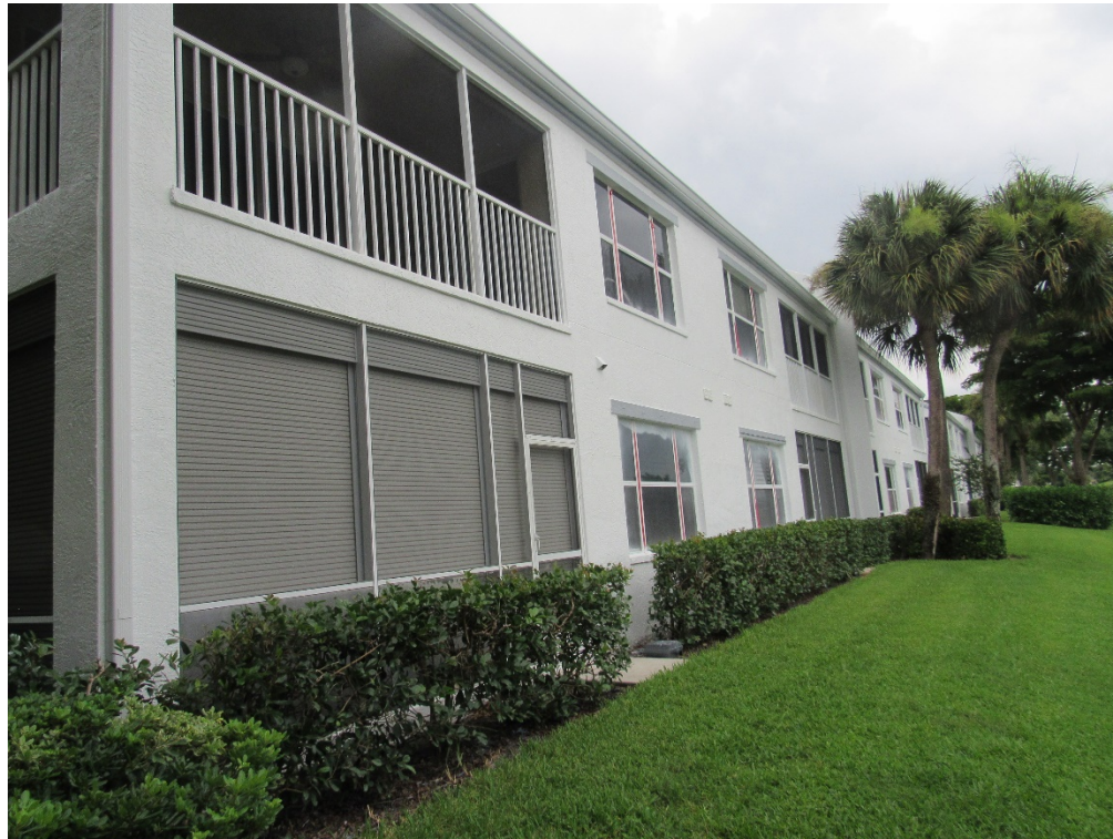
View of typical glazed openings (per question 7).
