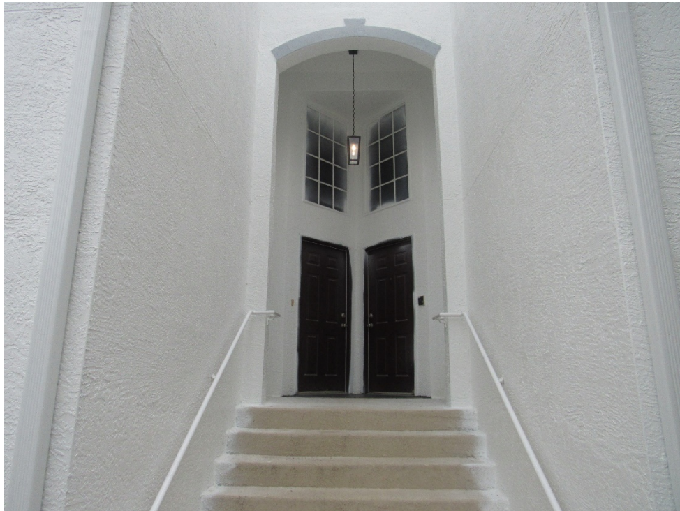
View of typical non-glazed openings (per question 7).
