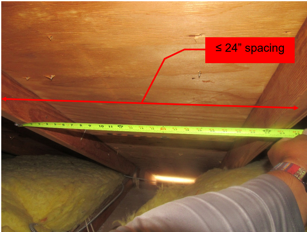
View of truss spacing (per question 3).
