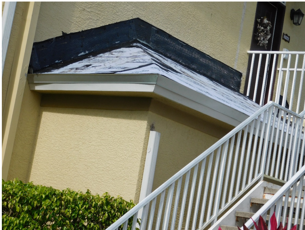
View of self-adhering roofing underlayment (per question 6).
