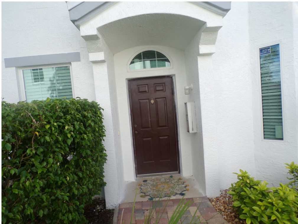
View of non-glazed openings (per question 7).
