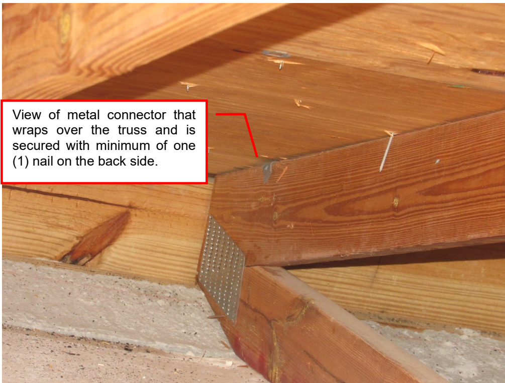
View of metal connector used on Roof to Wall attachment (per question 4).
