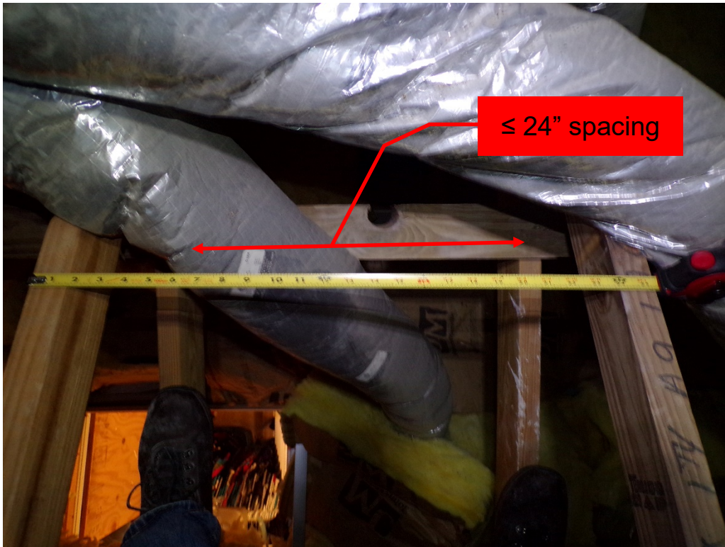
View of truss spacing (per question 3).
