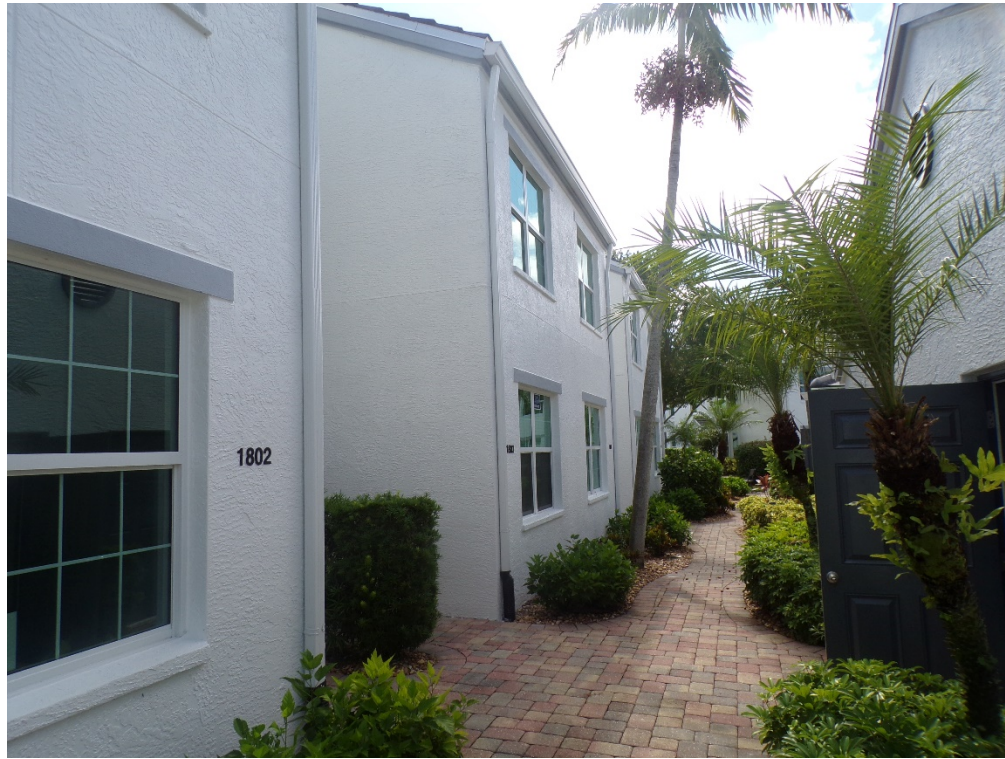
View of typical glazed openings (per question 7).
