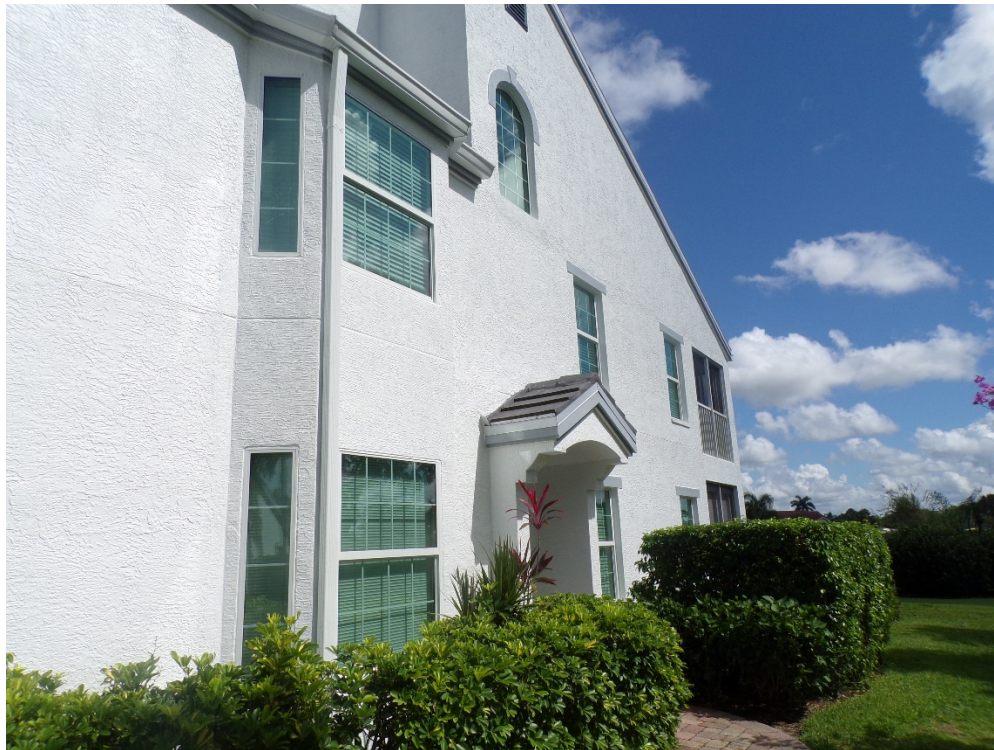
View of typical glazed openings (per question 7).
