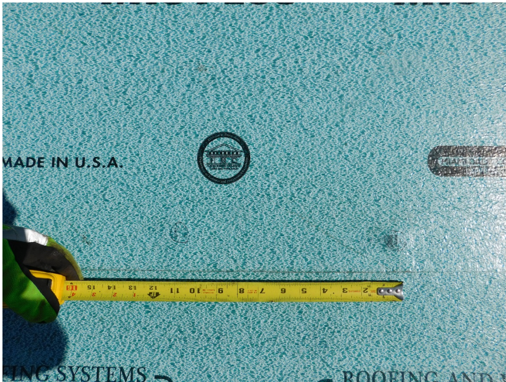
View of self-adhering roofing underlayment (per question 6).
