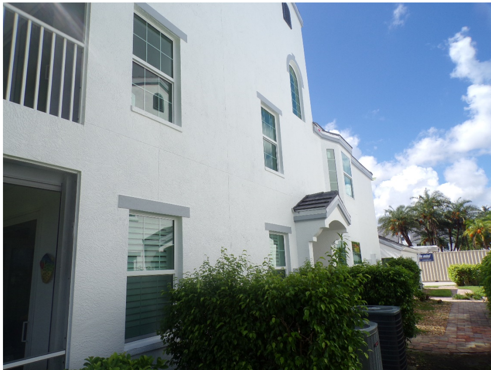
View of typical glazed openings (per question 7).
