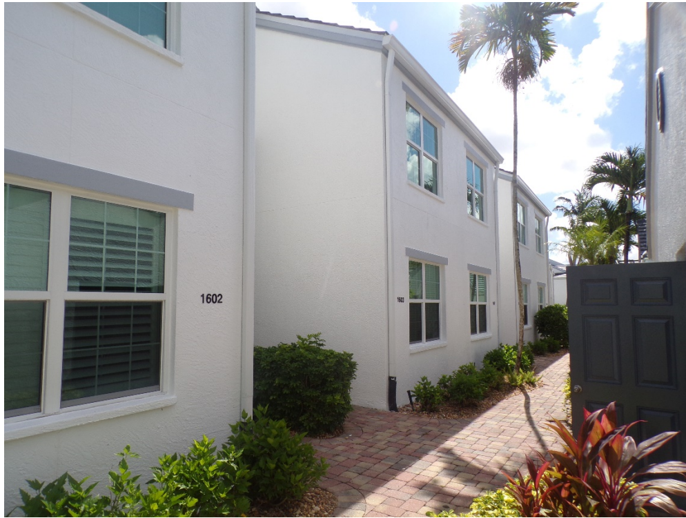
View of typical glazed openings (per question 7).
