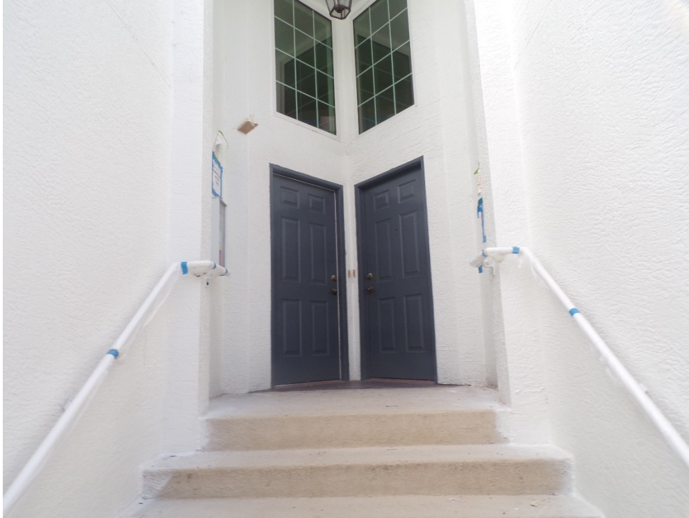
View of non-glazed openings (per question 7).
