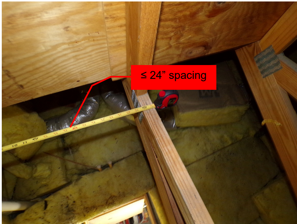
View of truss spacing (per question 3).
