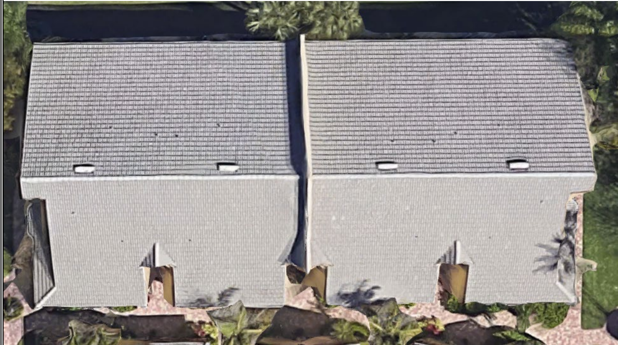
View of roof geometry (per question 5).
