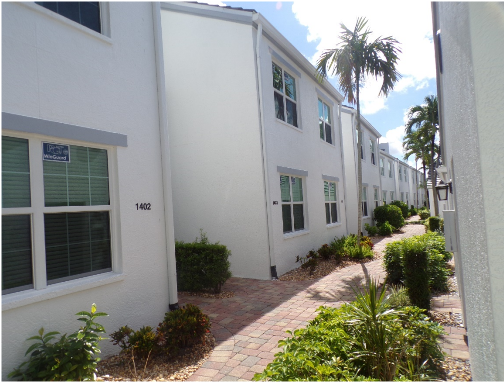
View of typical glazed openings (per question 7).
