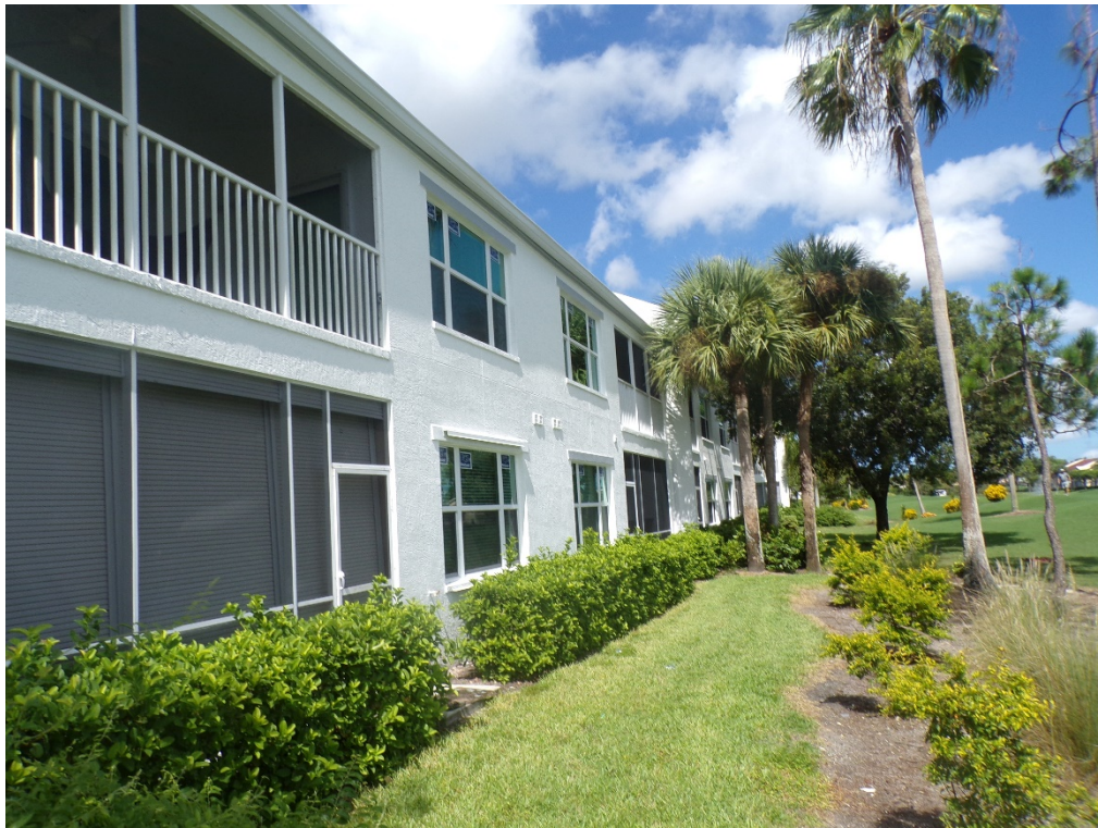
View of typical glazed openings (per question 7).
