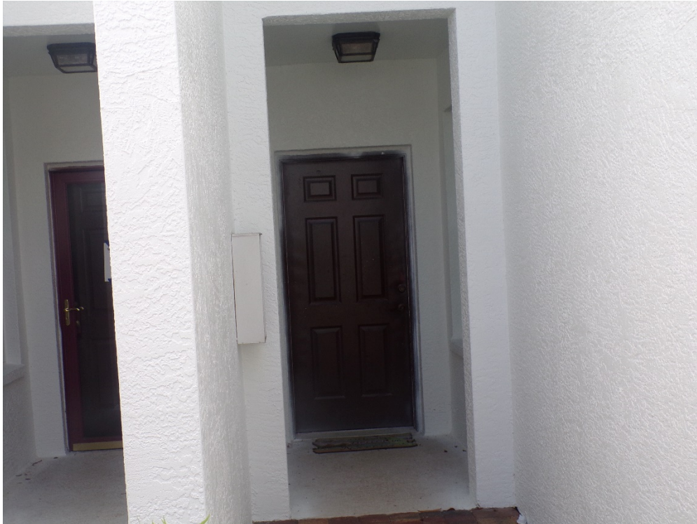
View of non-glazed openings (per question 7).
