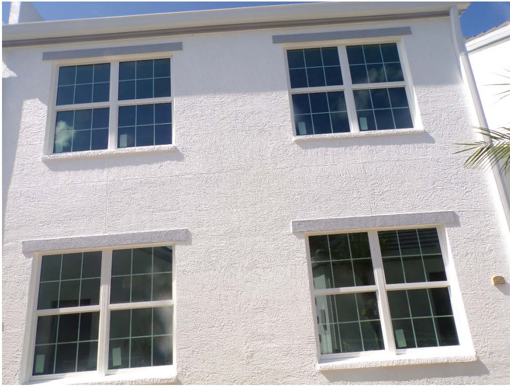
View of typical glazed openings (per question 7).
