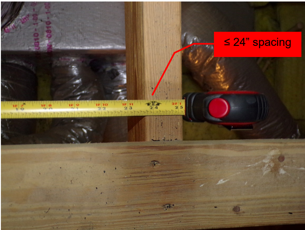
View of truss spacing (per question 3).
