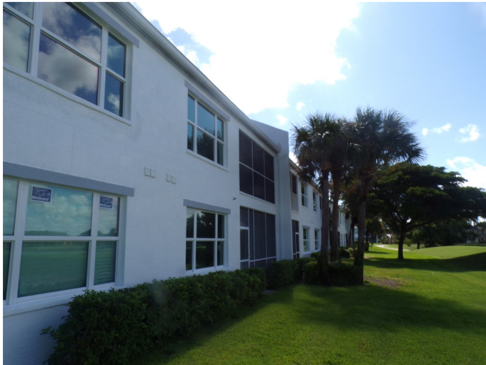
View of typical glazed openings (per question 7).
