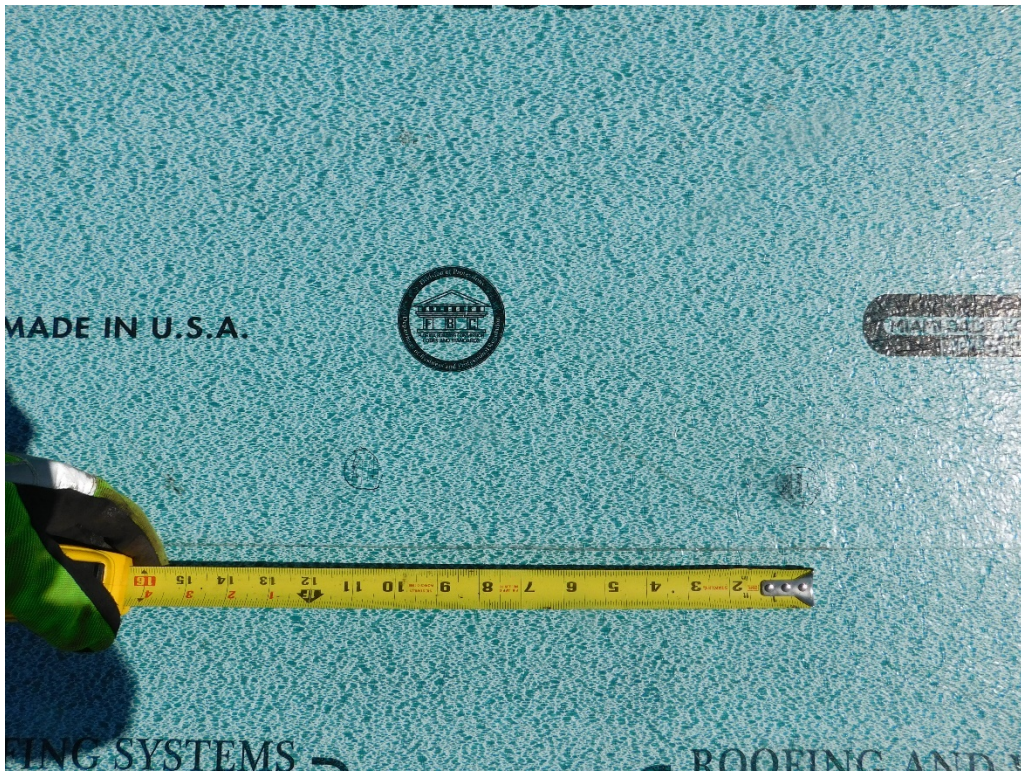
View of self-adhering roofing underlayment (per question 6).
