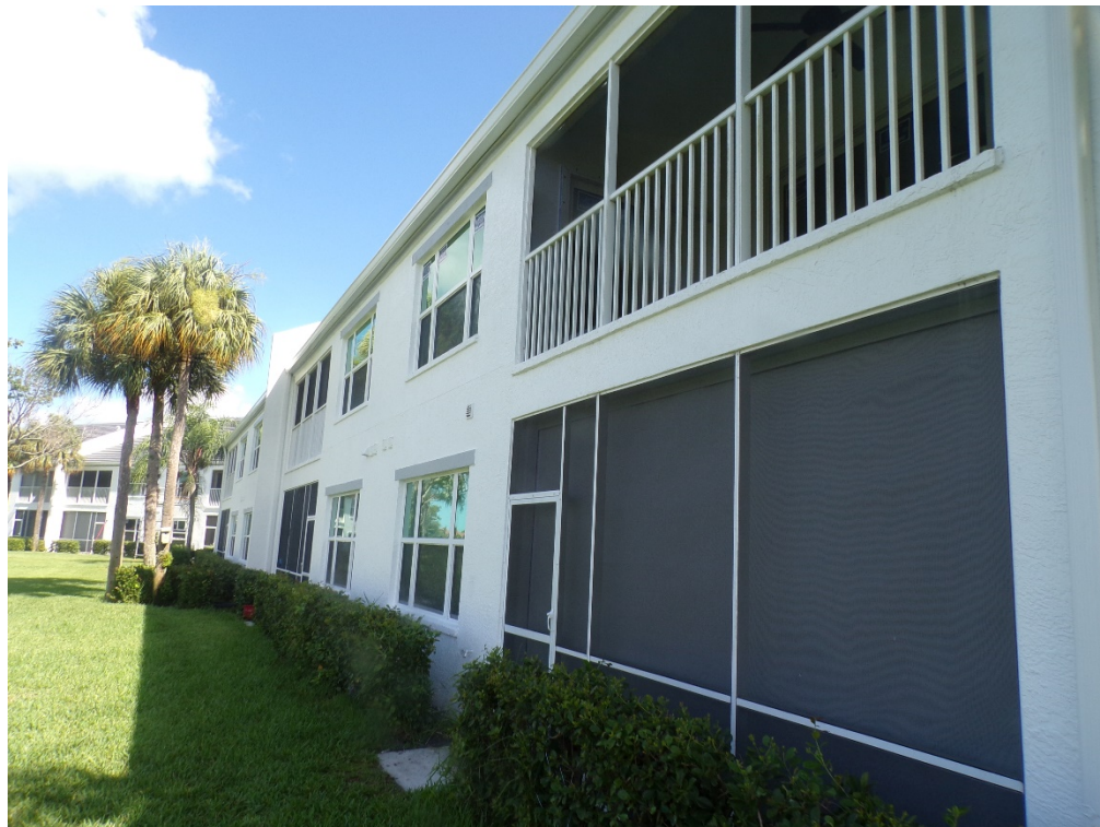
View of typical glazed openings (per question 7).
