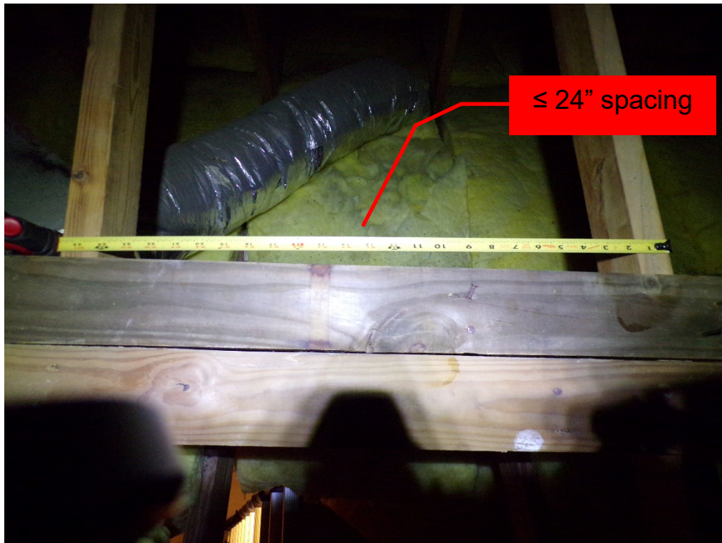
View of truss spacing (per question 3).
