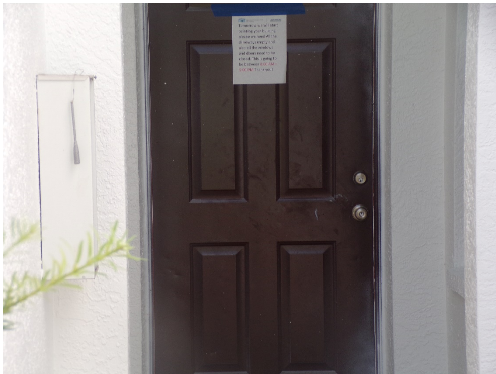
View of non-glazed openings (per question 7).
