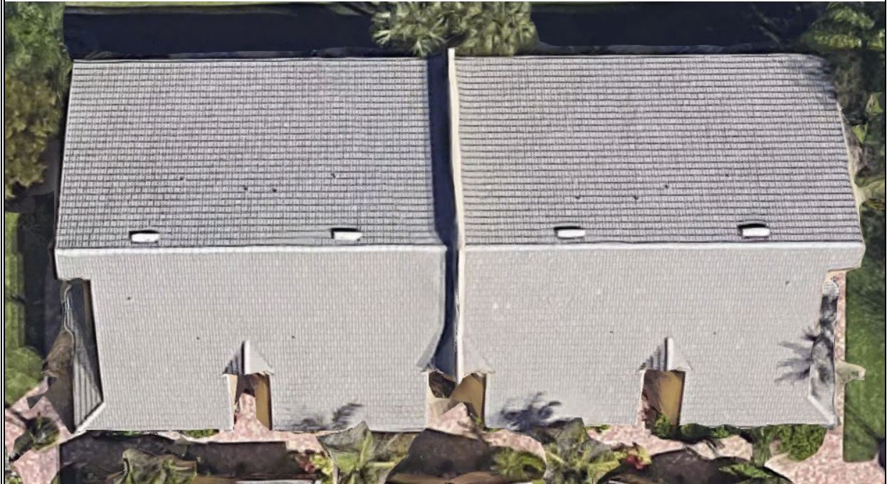
View of roof geometry (per question 5).
