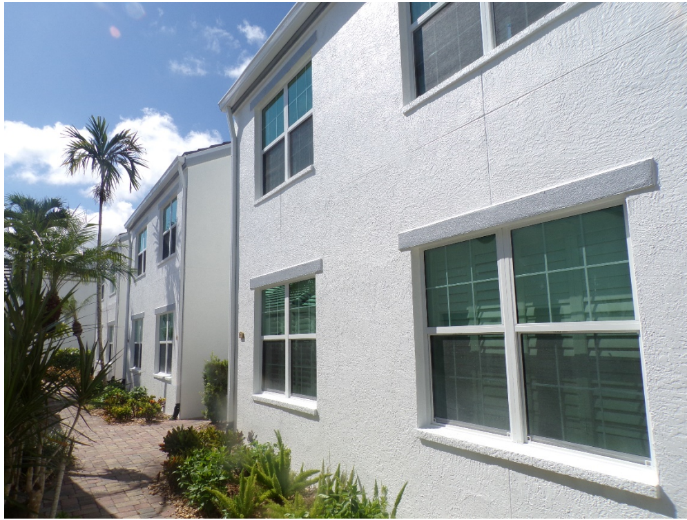
View of typical glazed openings (per question 7).
