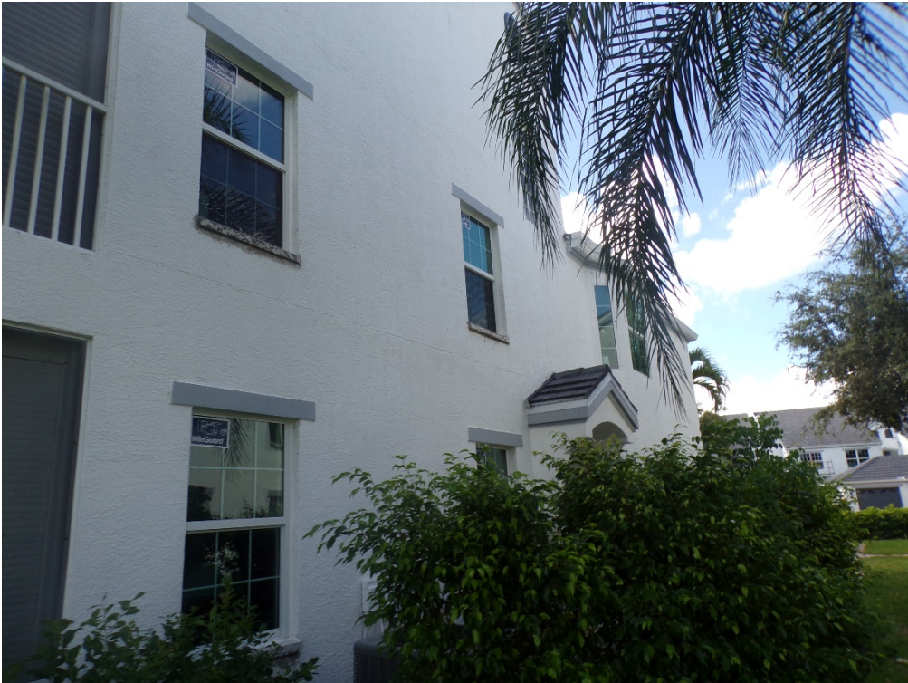
View of typical glazed openings (per question 7).
