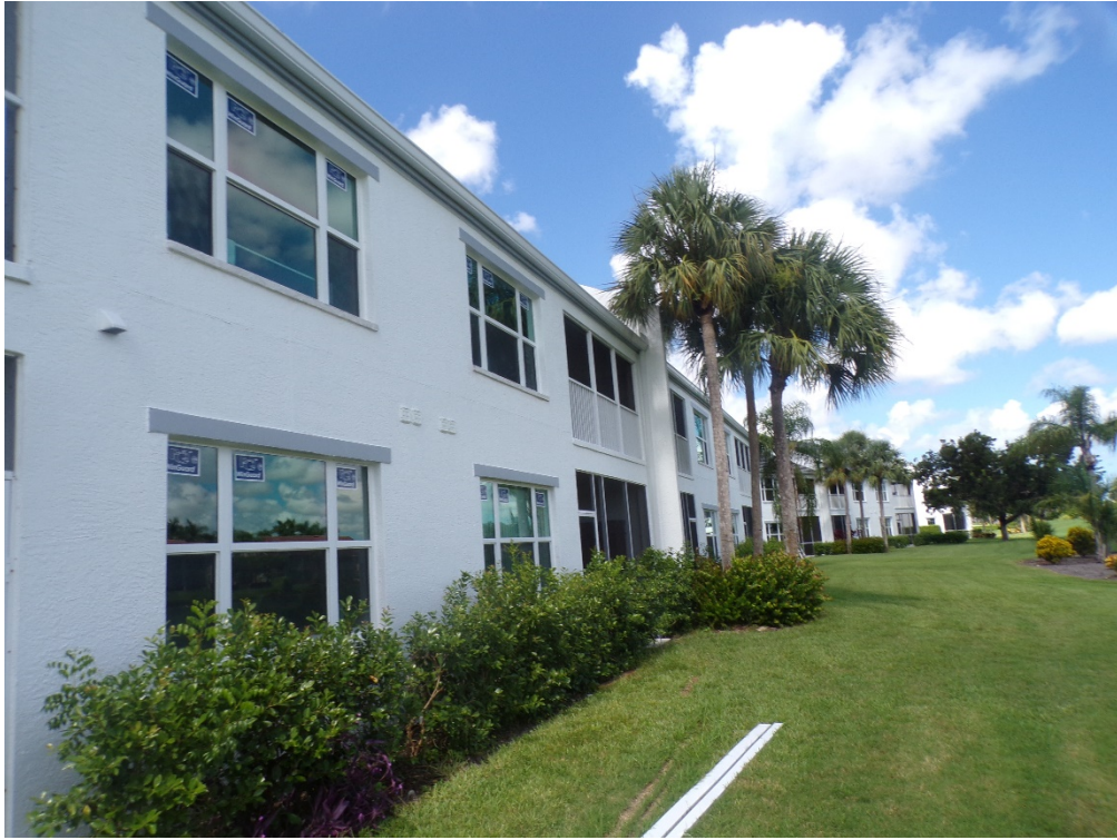
View of typical glazed openings (per question 7).
