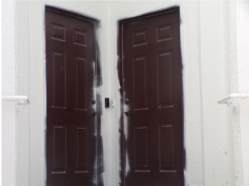
View of non-glazed openings (per question 7).
