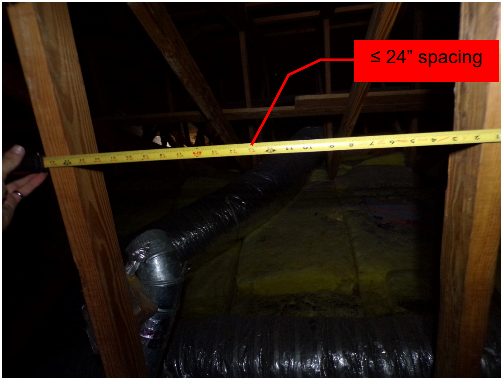
View of truss spacing (per question 3).
