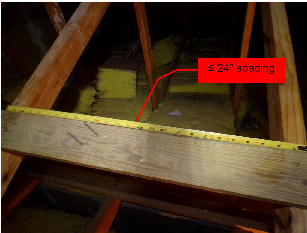
View of truss spacing (per question 3).
