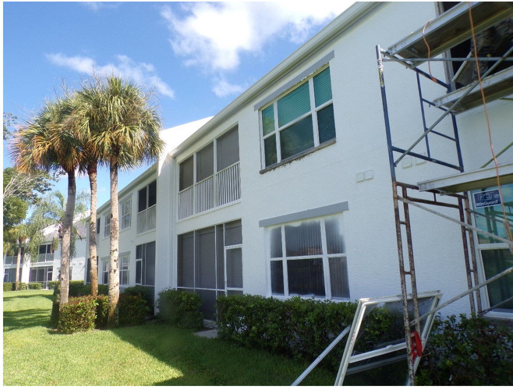
View of typical glazed openings (per question 7).
