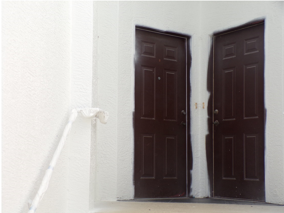
View of non-glazed openings (per question 7).
