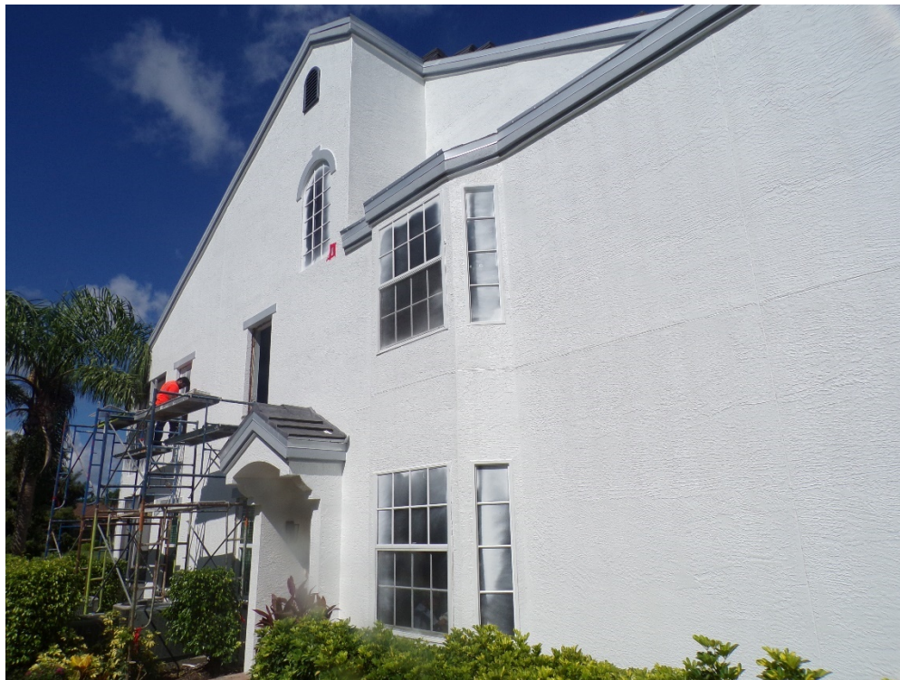
View of typical glazed openings (per question 7).
