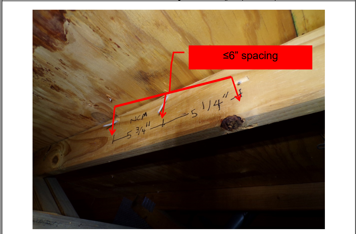
View of re-nailing pattern (per question 3).
